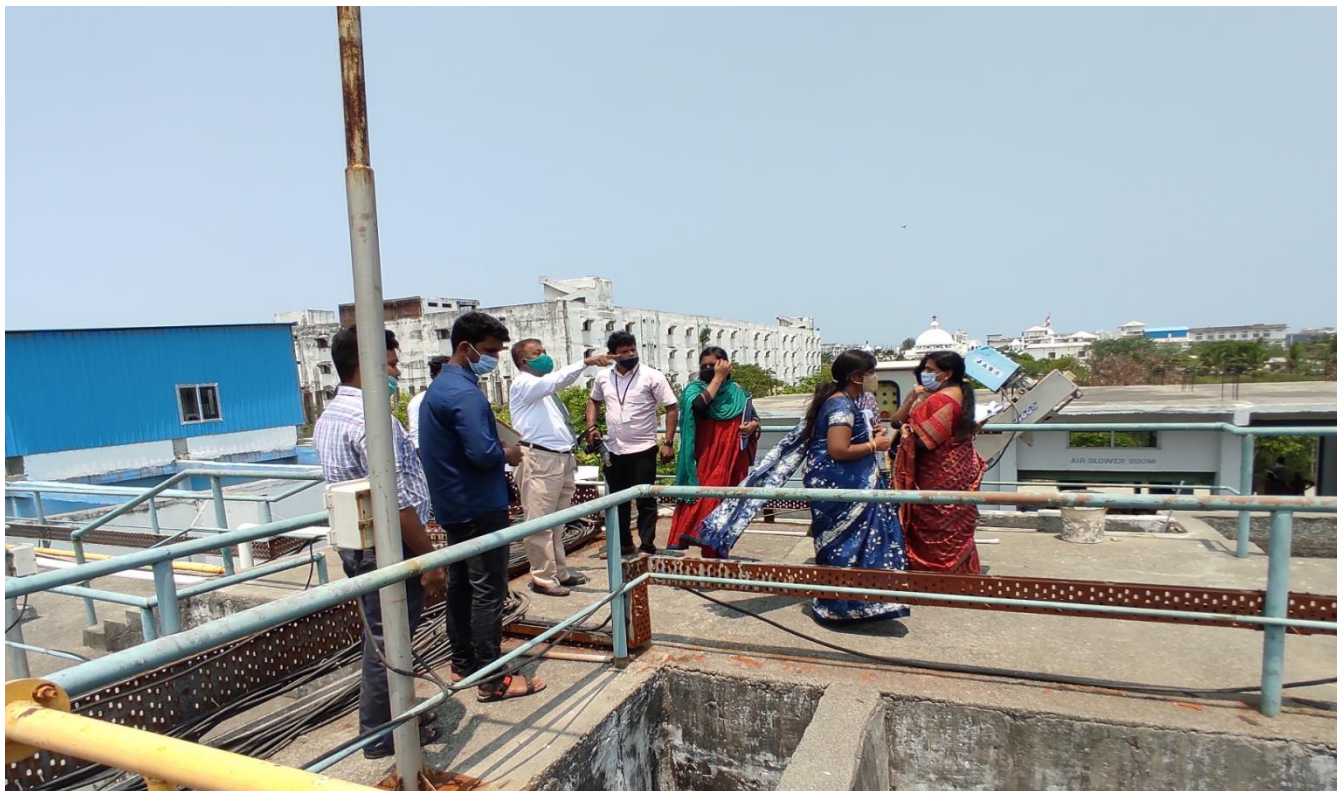
Figure 40: Audit Team visits the STP
