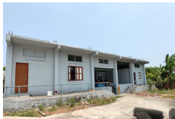
Figure 13: Control Panel Rooms
