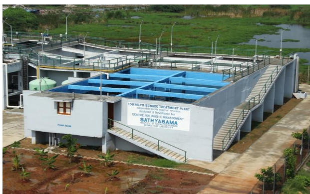
Figure 12: STP Plant Overview
