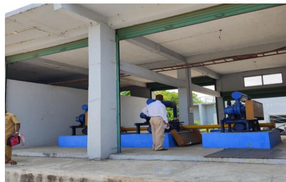
Figure 11: Site visit at STP
