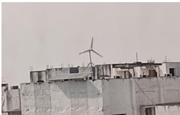
Figure 14: Solar-Wind Hybrid system at the institute
