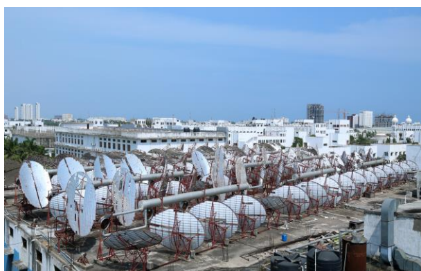
Figure 16: Solar Powered Cooking System
