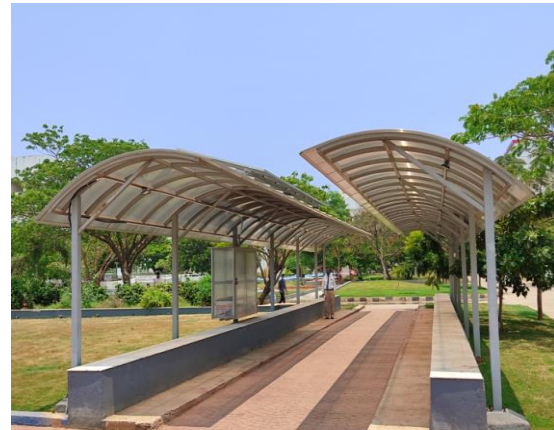
Figure 38 : Solar roofed sitting area
