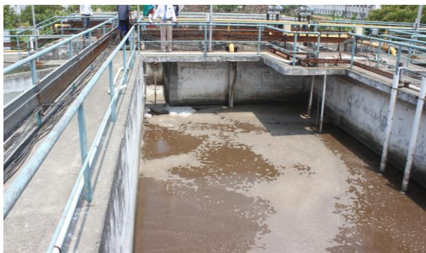
Figure 10: Sewage treatment plant
