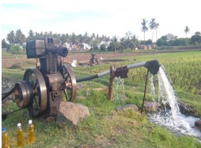
Figure 23: Biodiesel developed from waste cooking oil used to run Generator
