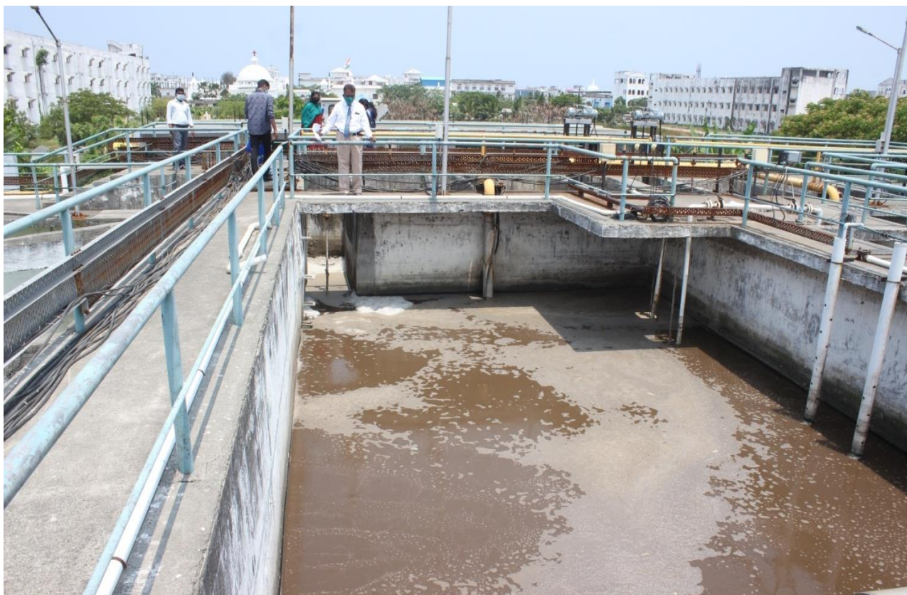
Figure 32: STP-SBR-Unit
