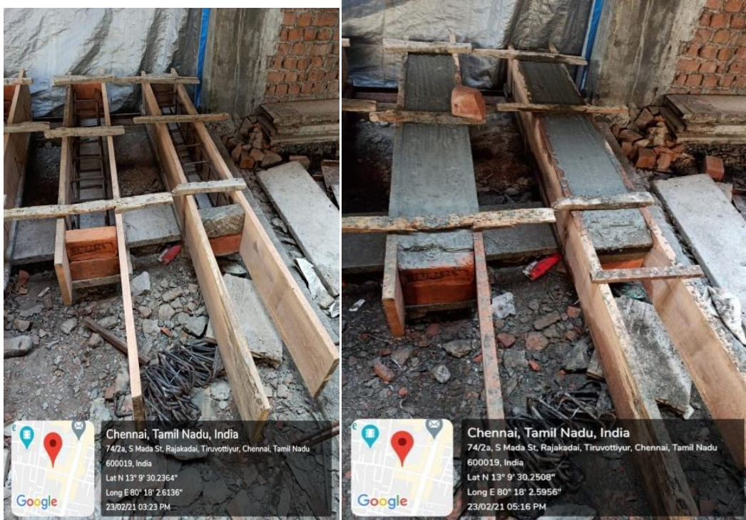
Fig.4.7. RC Beam Casting
