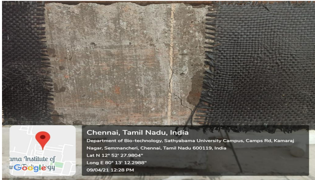
Fig 5.6 First crack on CFRP wrapped beam with 200 mm interval
