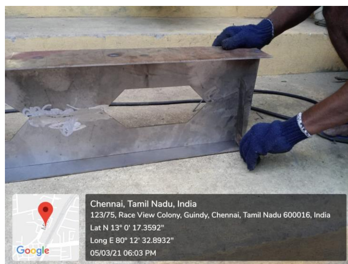
Fig 6.8: Arc Welding of Beams
