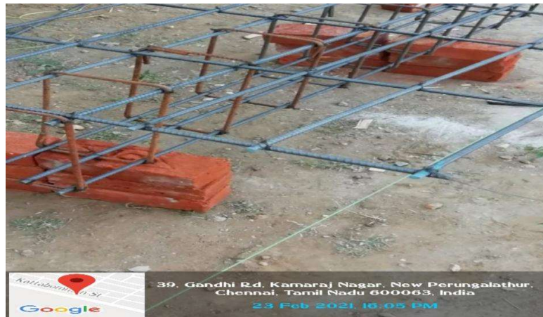
FIG 4.3 REINFORCEMENT FOR CASTING OF BEAM
