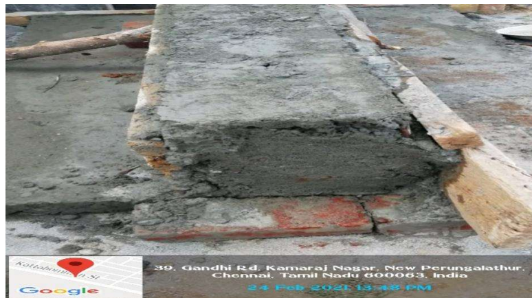
FIG 4.4 CASTING OF BEAM
