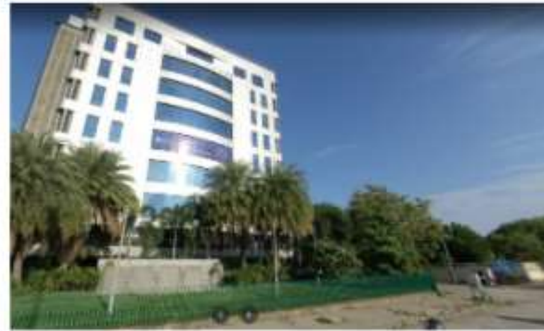
IT building in perungudi near the proposed site for metro
