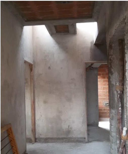
Filler slab roof
