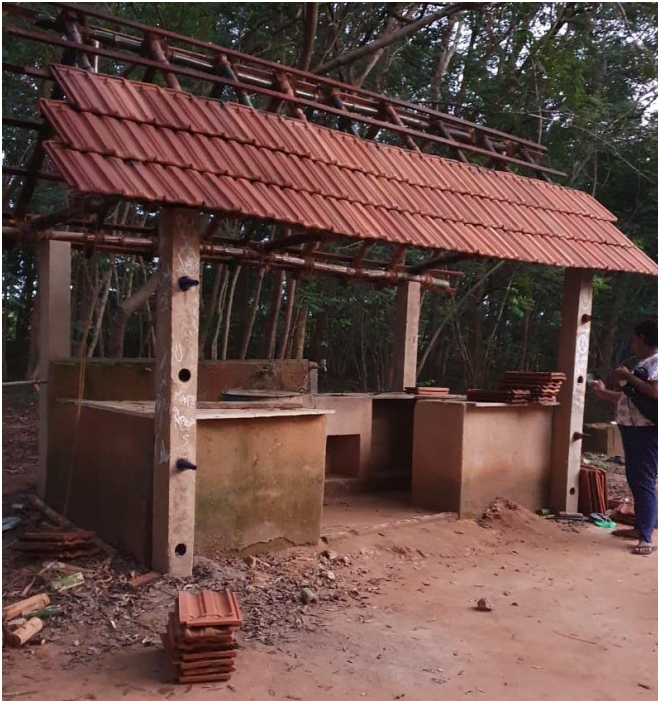
Bubble Area After Laying Terracotta Tiles
