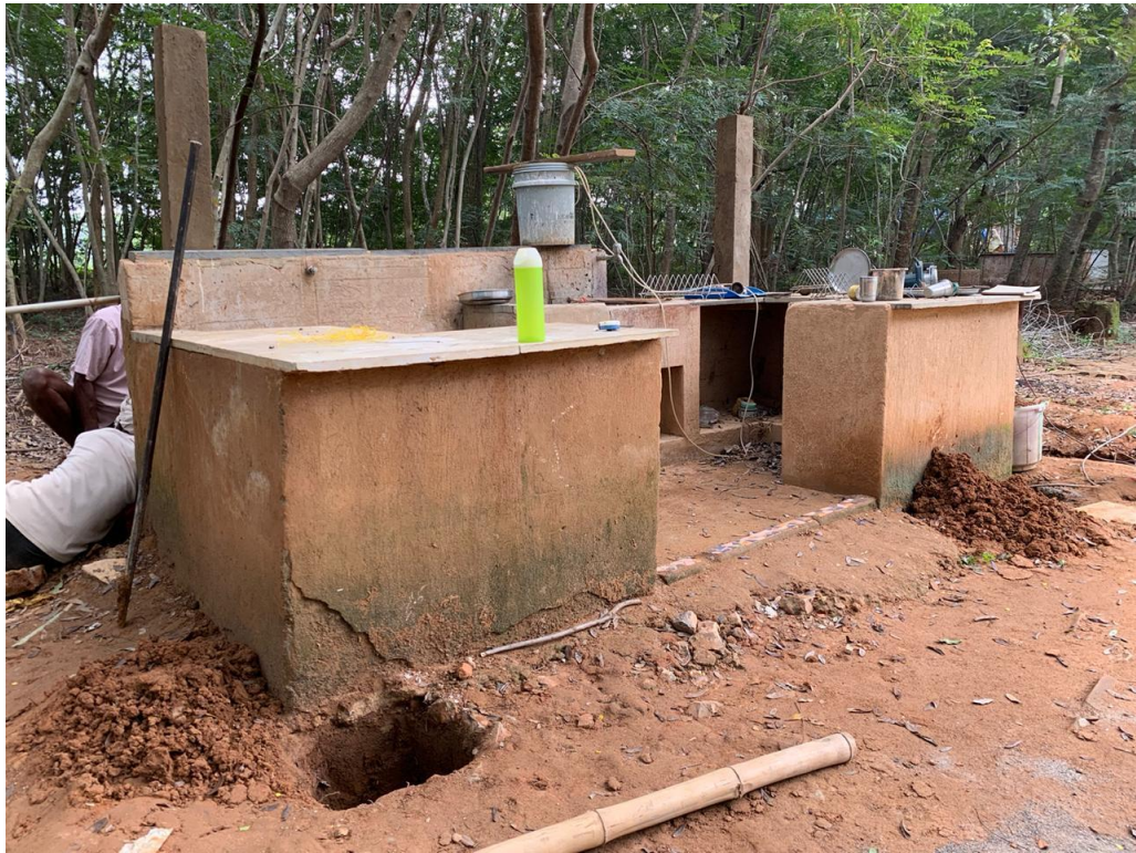
Tubular Level for Checking the levels of all the 4 columns without any height difference.
