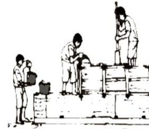
POURING THE MIX INSIDE THE FORMWORK
