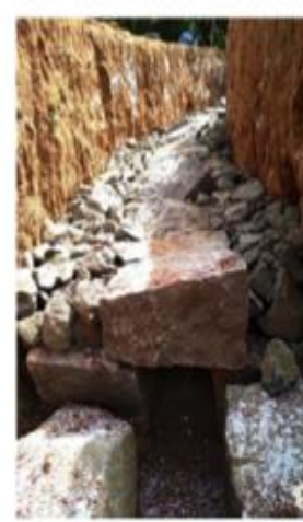
RUBBLES LAD VERTICAL , WITH THE GAP OF 4" IN BTWN THE SIDE WALLS OF CHANNEL
