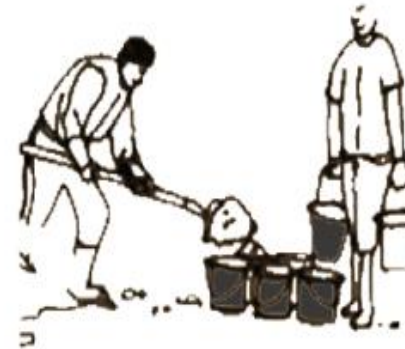
SHIFTING THE MIX
