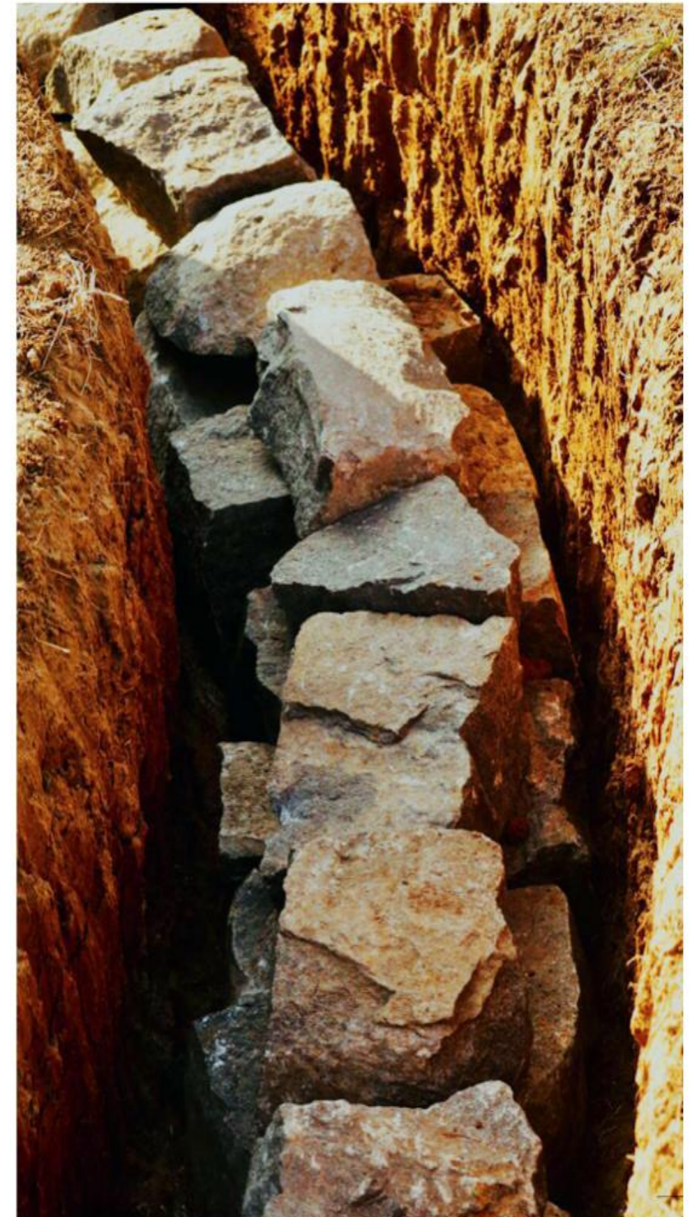
RUBBLES LAD VERTICAL , WITH THE GAP OF 4" IN BTWN THE SIDE WALLS OF CHANNEL
