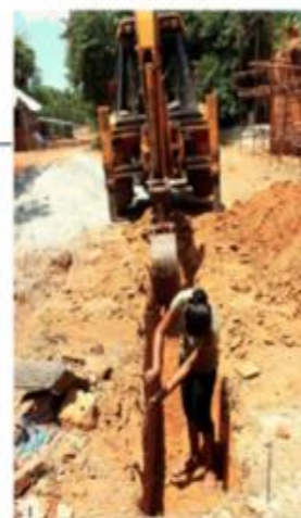
DIG THE TRENCH WITH THE DROP OF 1CM FOR EVERY 1M
