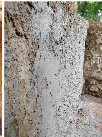
Palingu Plastering
