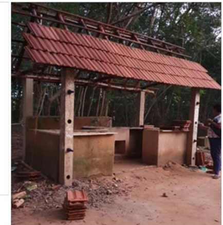
Bubble Area After Laying Terracotta Tiles
