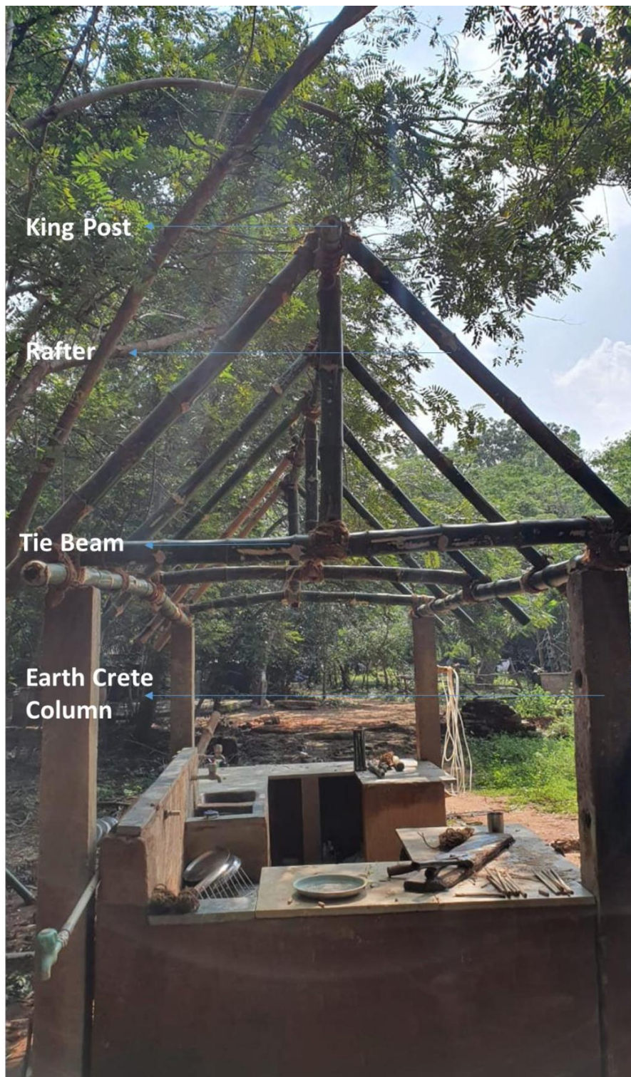
Bamboo Lashing with coir rope Japanese Square Lashing technique
