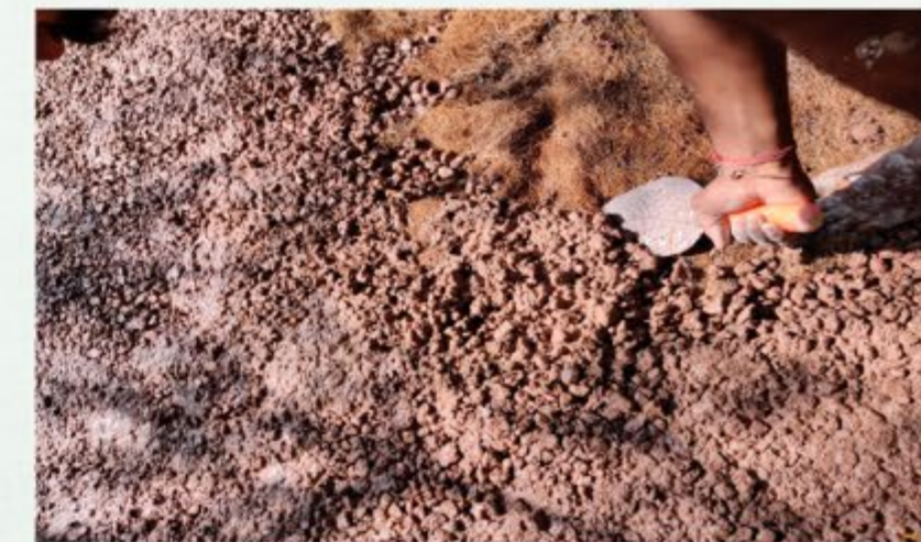
EARTHCRETE ON ROOF
