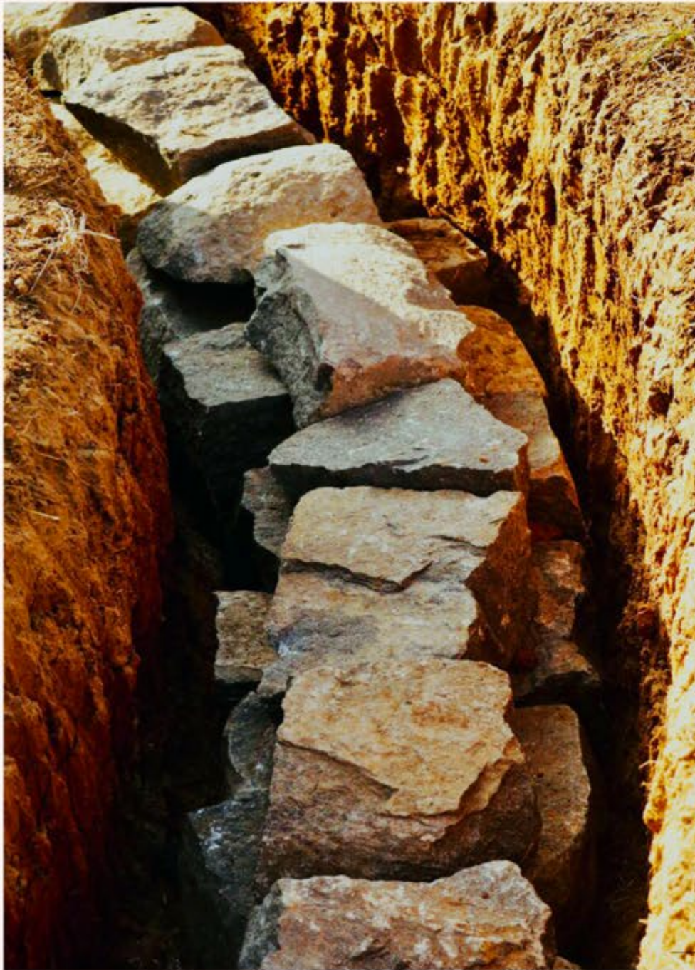
Rubble masonry foundation
