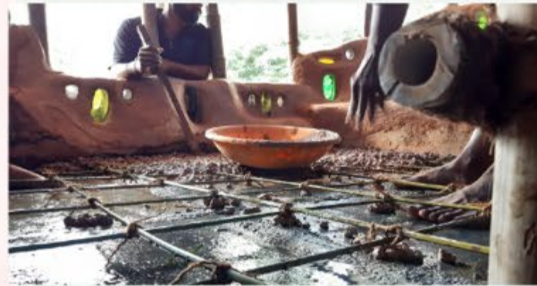
REINFORCEMENT ON MEZZANINE
