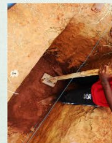
THE DIG TRENCH IS LEVELLED ACORDING TO SLOPE
