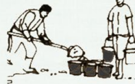
SHIFTING THE MIX
