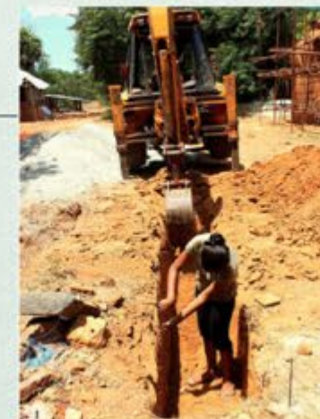
DIG THE TRENCH WITH THE DROP OF 10MM FOR EVERY 1M
