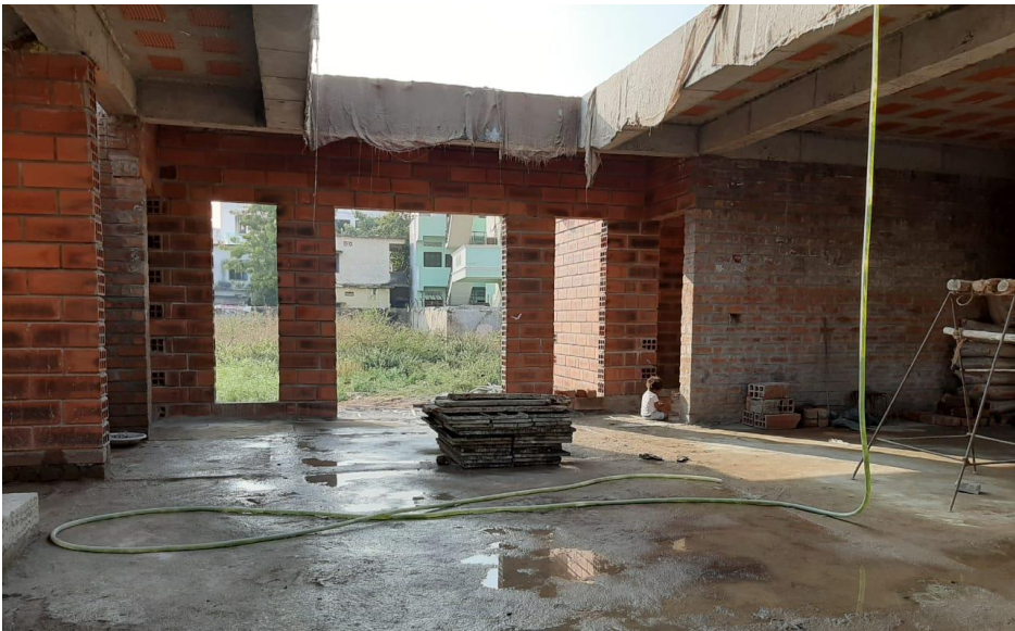
Hollow clay block arch
