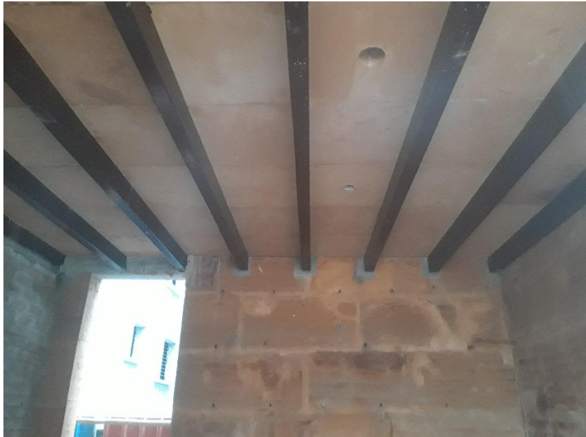
Rammed earth roof
