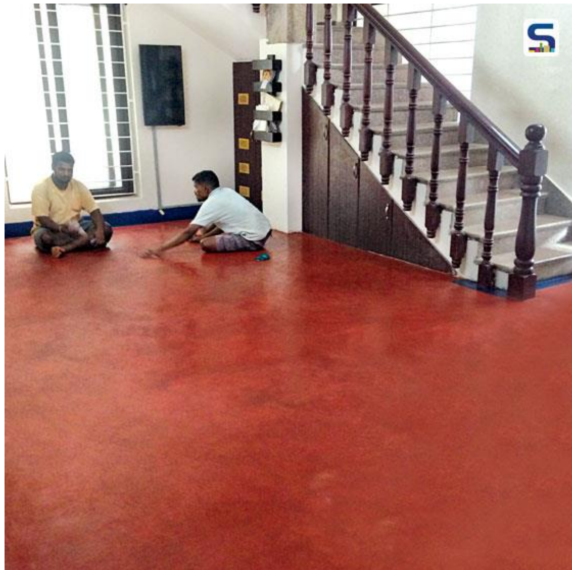
Image 3- Shows how red oxide flooring be manually done on the floor of residence.
