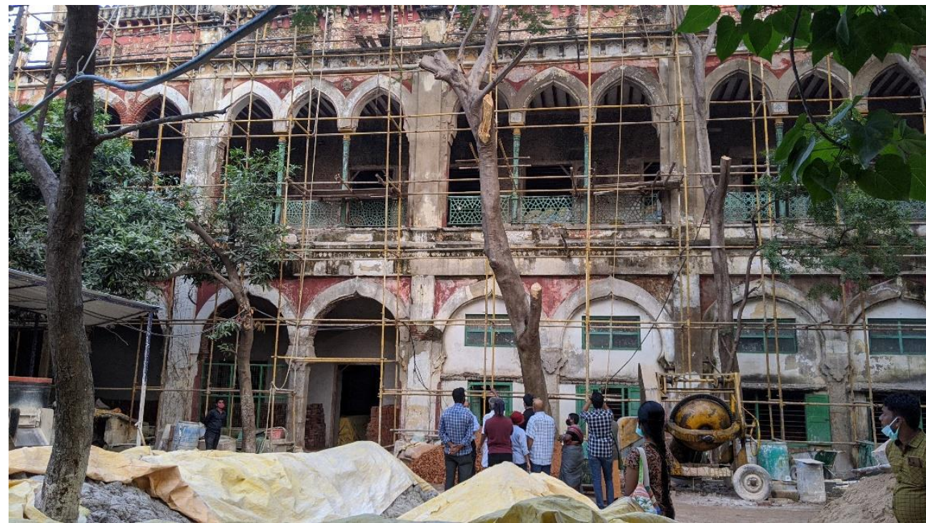
Image 4-the space back side of the building used for preparing and storing lime
