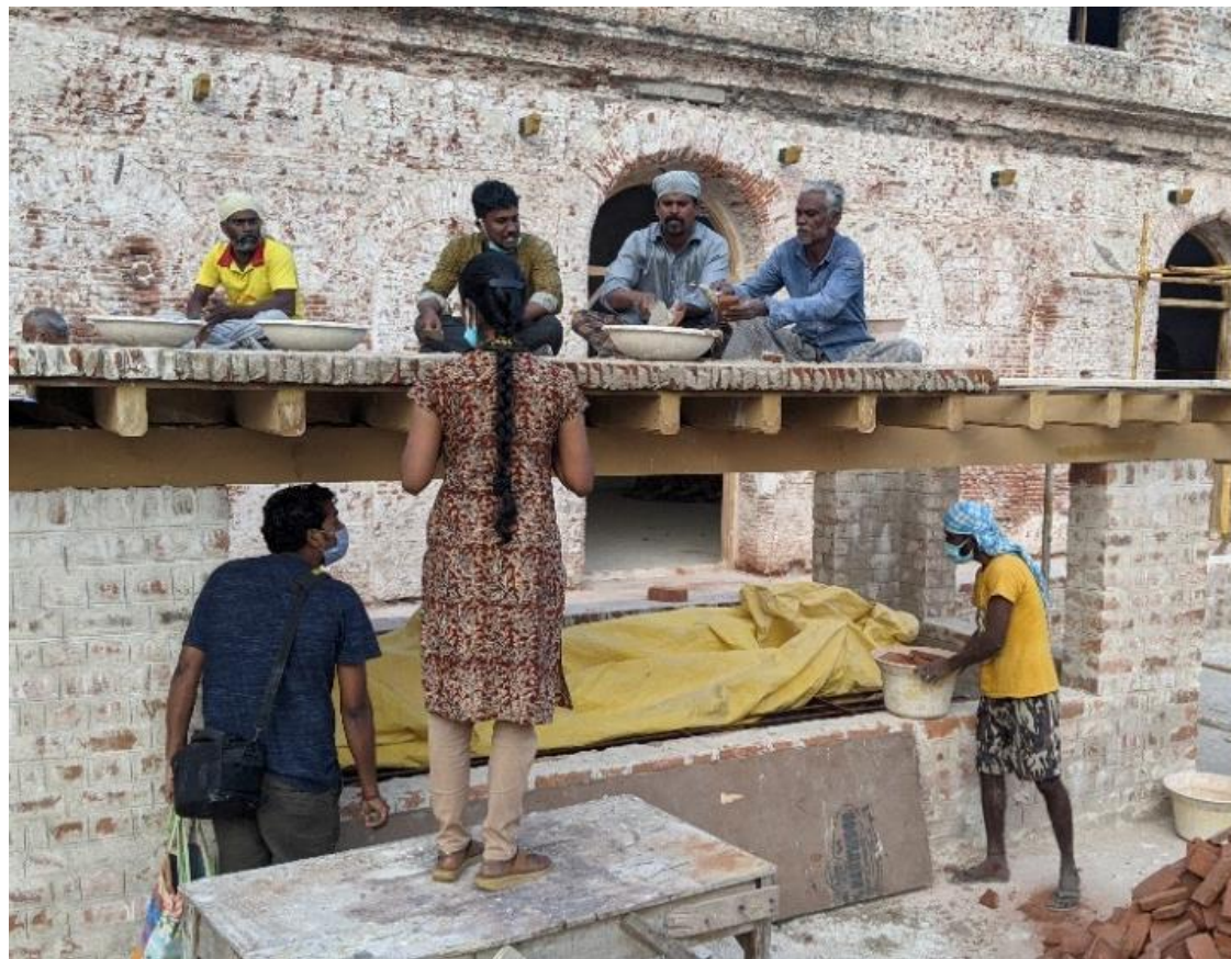
Image 9-craftsmen demonstrating the construction of madras terrace roofing
