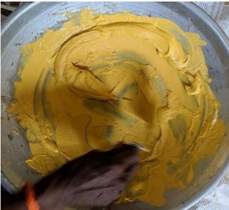
Image 1- Shows mix of lime plaster cement with colored oxide.
