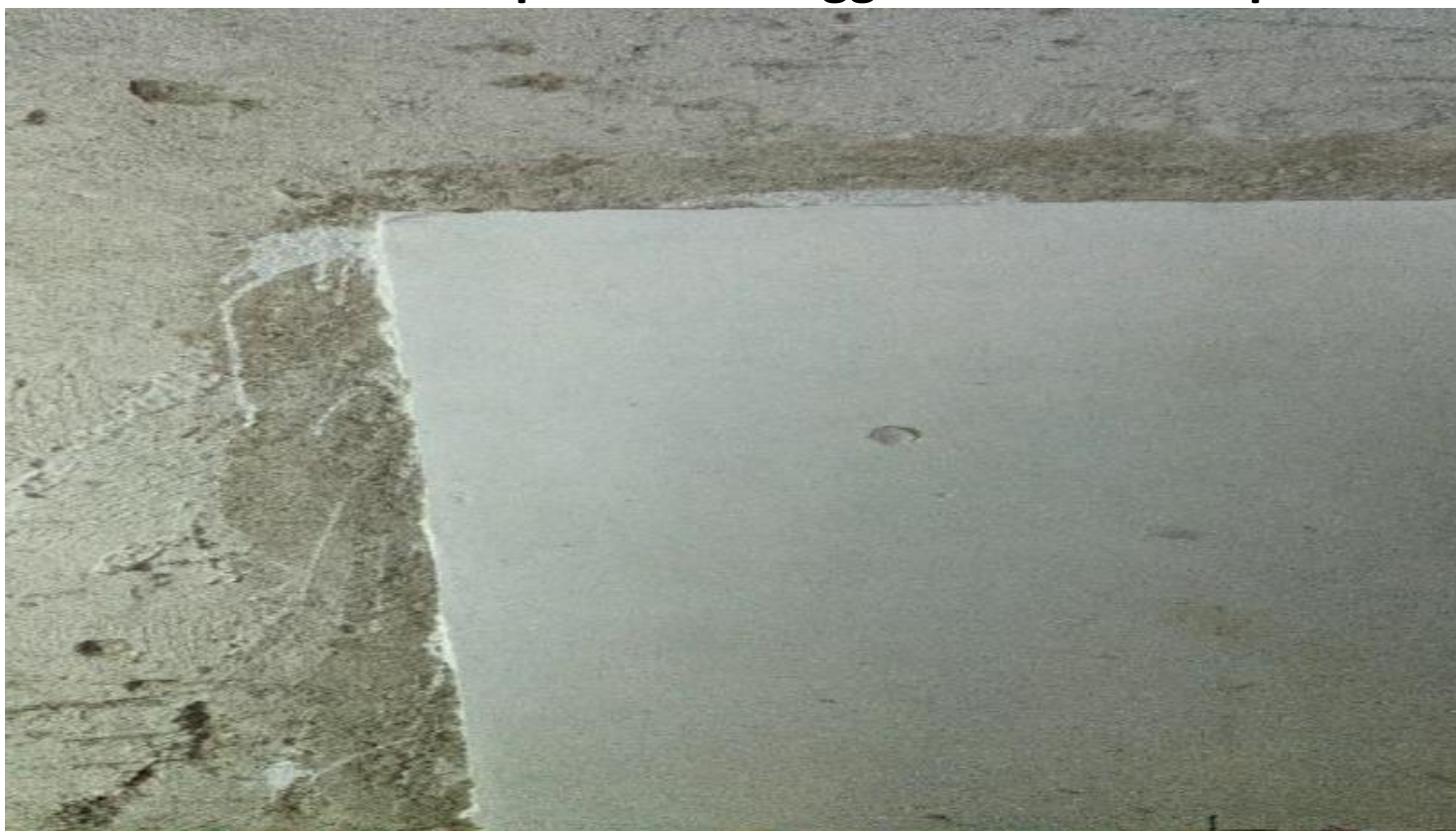
Image 7- sample of finished Mughal plastering
