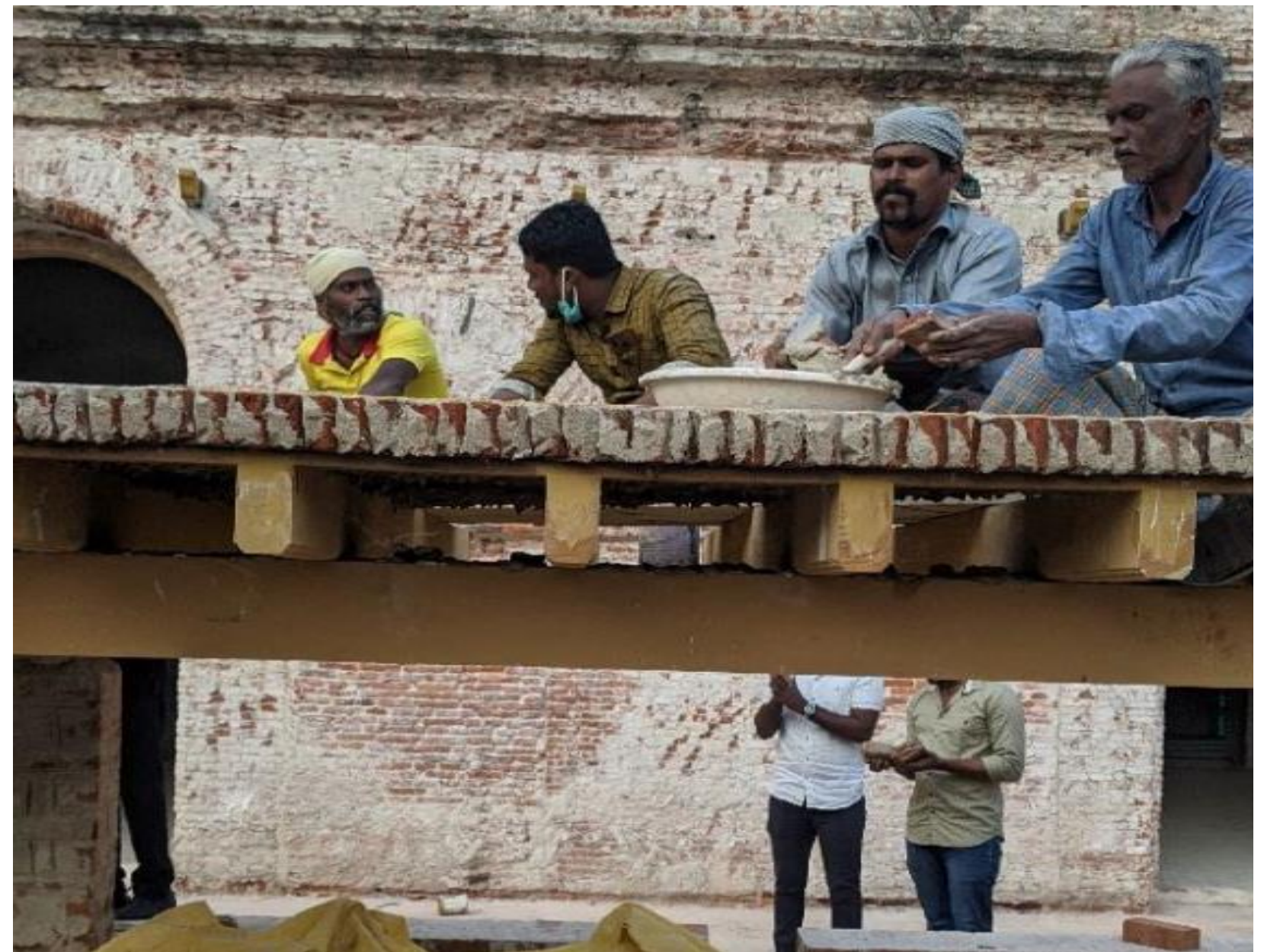
Image 9-craftsmen demonstrating the construction of madras terrace roofing
