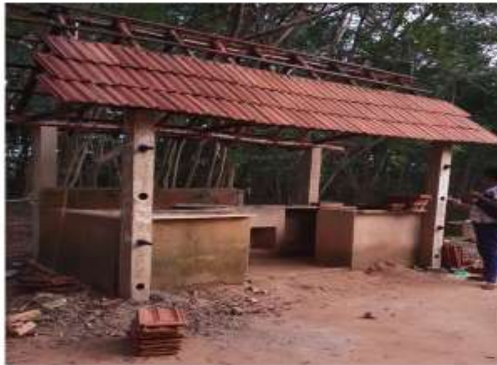
After placing mangalore tiles
