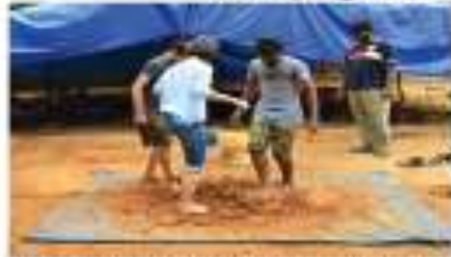
The mix of earth, rice husk & water well stamped and kneaded
