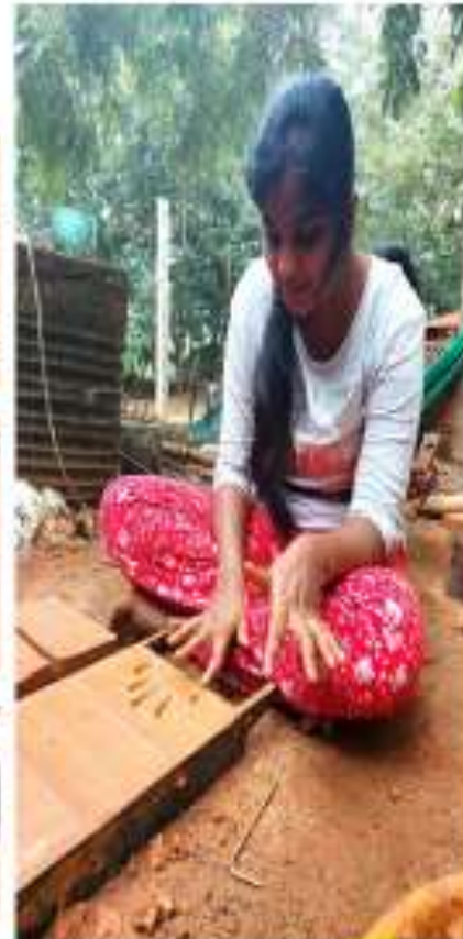
The mix of earth, rice husk & water well stamped and kneaded
