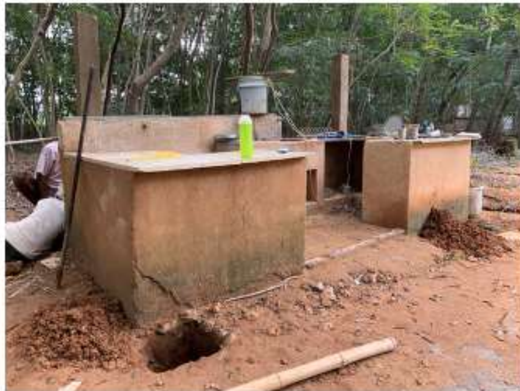
Dismantling of the structure and creating pits to at proper levels and measuring it with tubular level.
