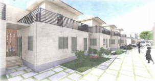
NORTH FACADE VIEW
