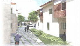
SOUTH FACADE VIEW
