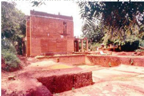
Fig: 2.2 Excavation of the basement floor – 1.2 m below the third building
