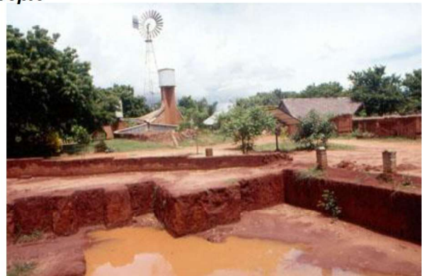
Fig: 2.2 Excavation of the basement ground level
