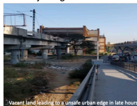
Vacant land leading to a unsafe urban edge in late hours
