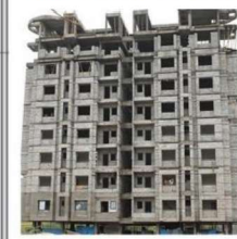
AAC block Construction
