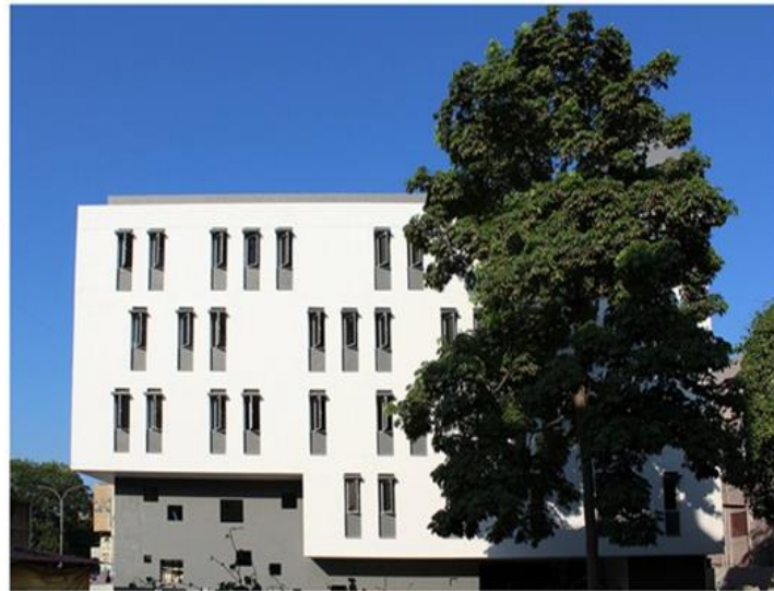
WESTERN FACADE : Slit windows at random patterns protect the Inside from the harsh-sun.
