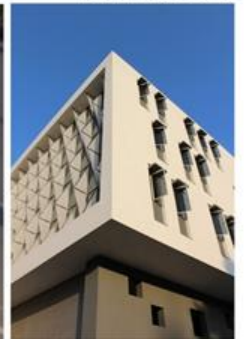
BUILDING ARTICULATION : S-West Facade
