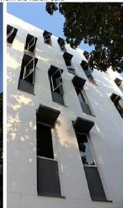
DESIGN : SLIT-WINDOWS:Effective Solution for West.
