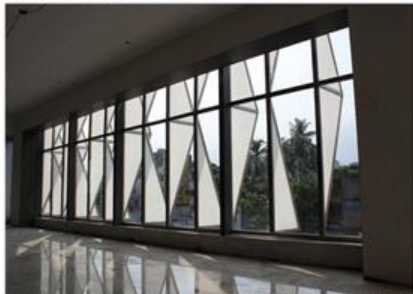
DAY-LIGHTING: The Northern Louvers create Glare-free Natural Light.
