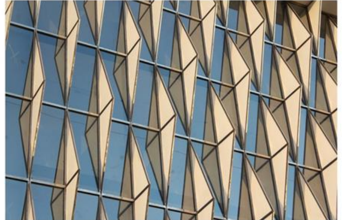
INNOVATIVE FACADE: Translucent shading devices designed to filter the Sun-light.
