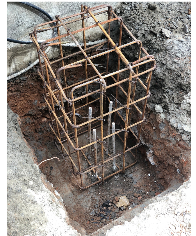
PILE FOUNDATION FOR LAMP POST
