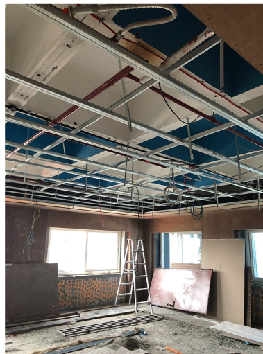
Fixage of Aluminium channels
