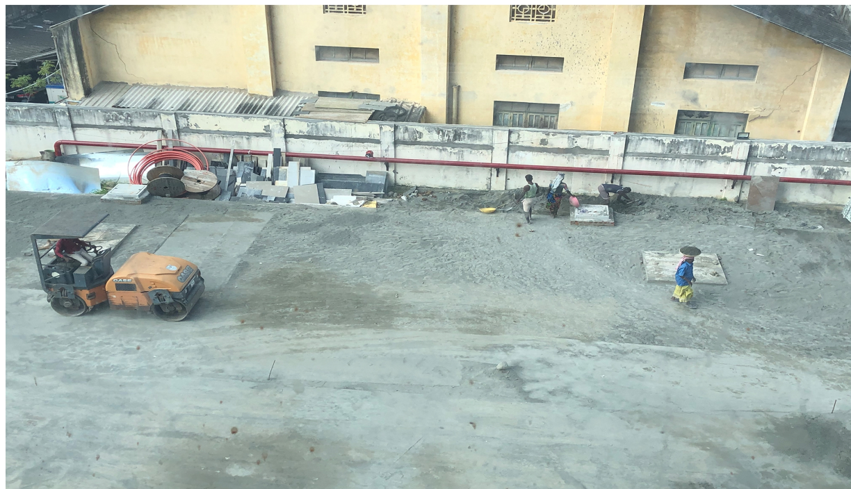
SITE LEVELLING AFTER SAND FILLING
