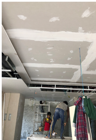
Gypsum Plaster Was done to make Joint free of two boards
