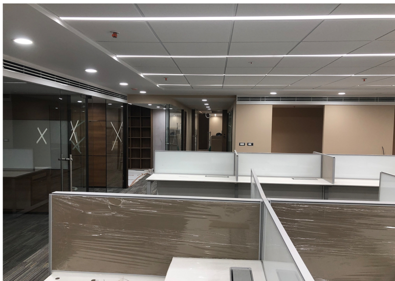
Post Installation Of Grid Ceiling
