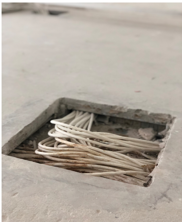
AFTER POURED CONCRETE SCREED FOR 2.5"
