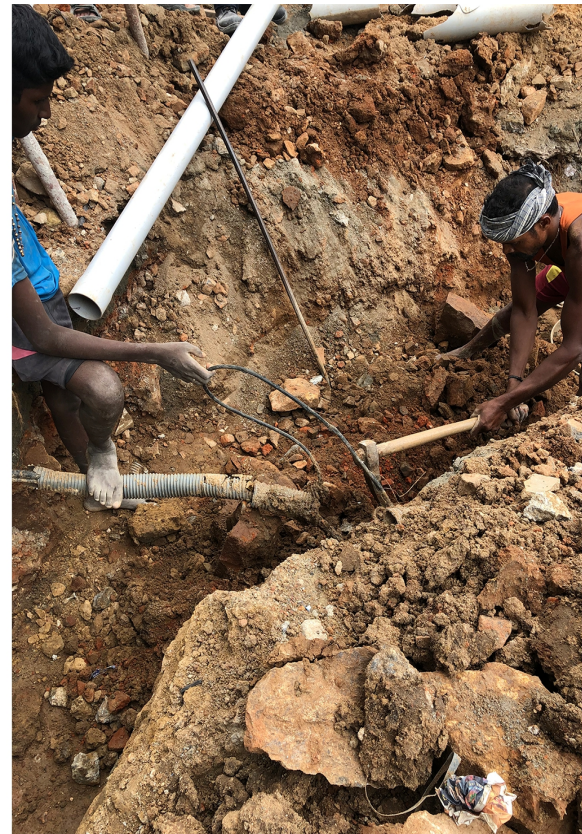
EXCAVATION FOR TRENCHES
