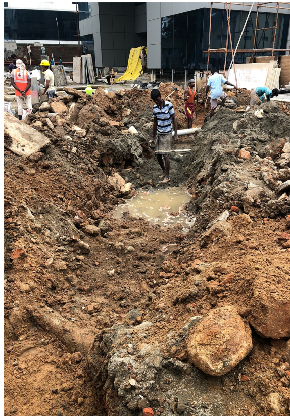
EXCAVATION FOR TRENCHES
