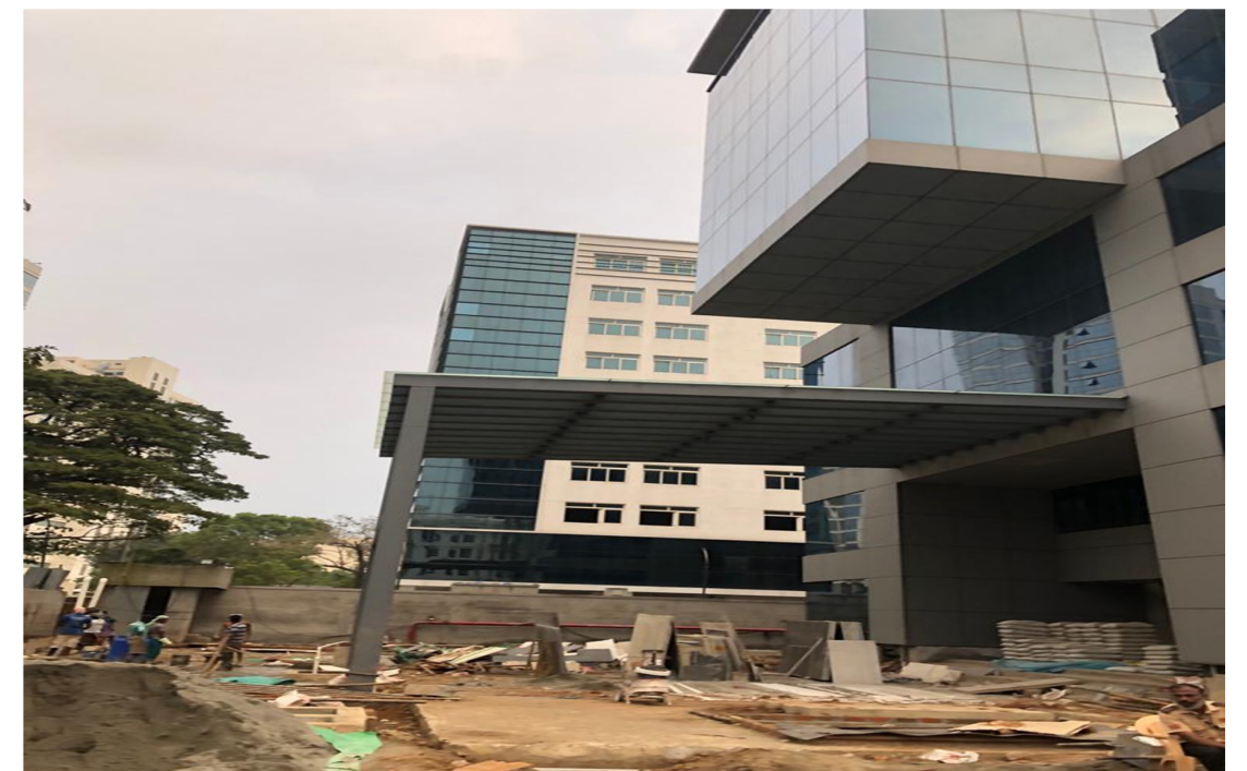
INFRASTRUCTURE WORKS ONGOING ON SITE
