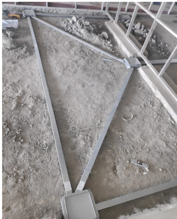
RACEWAYS LAYING
