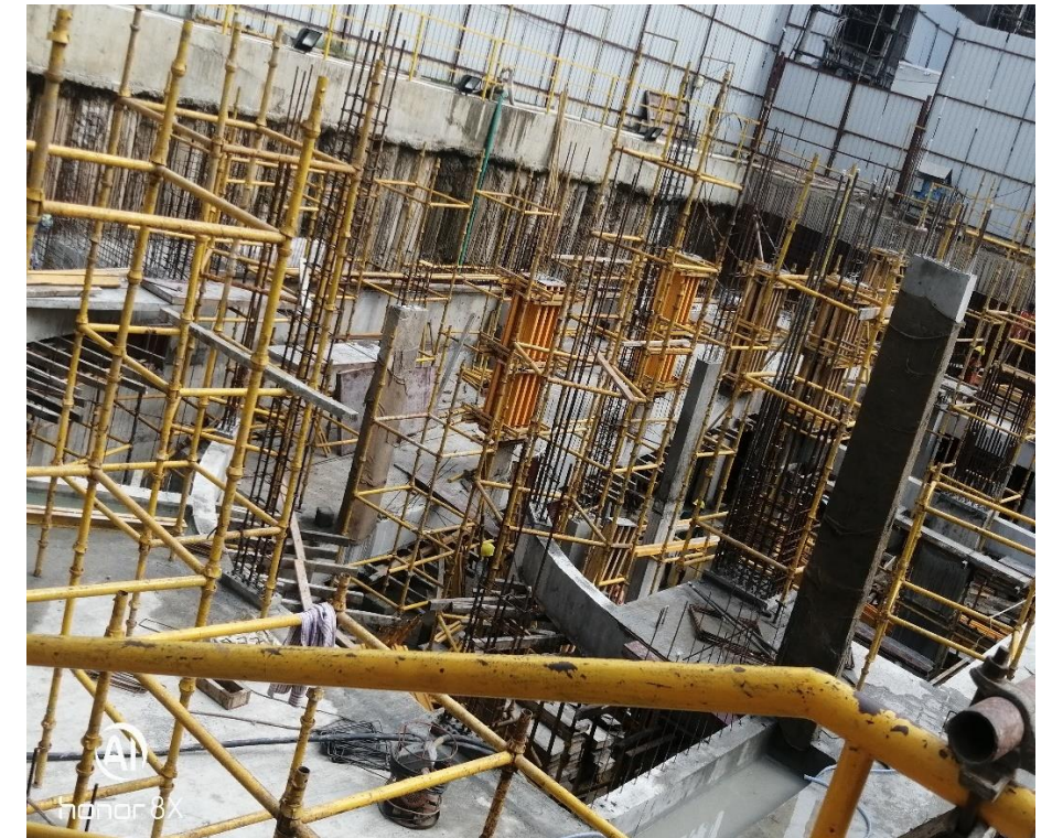
SUBSTRUCTURE UPTO BASEMENT
