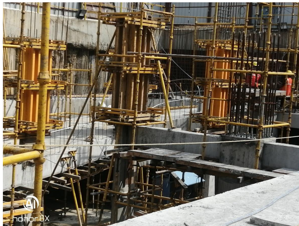
FORMWORK FOR BASEMENT COLUMN
