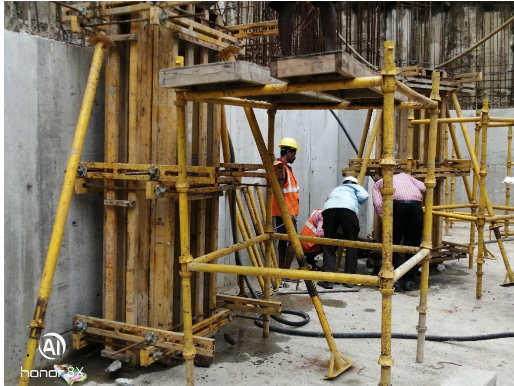
QUALITY TEST AFTER CONCRETING
