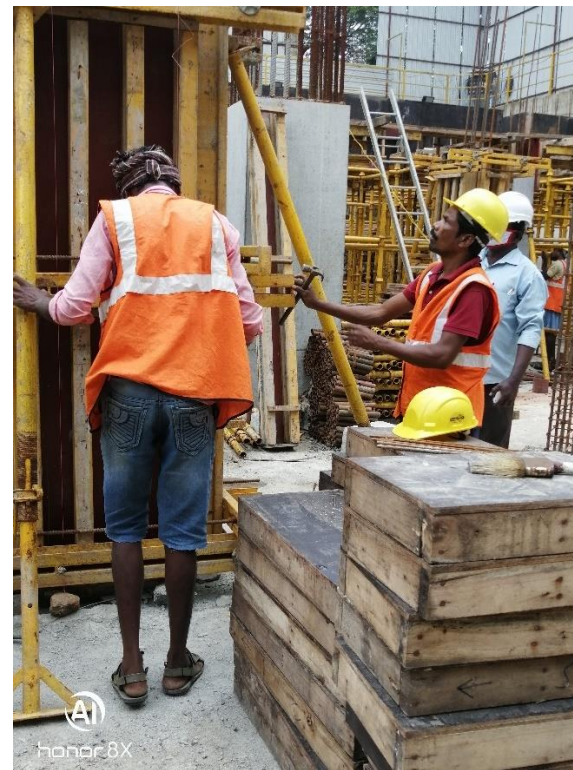
PROPPING FOR FORMWORK
