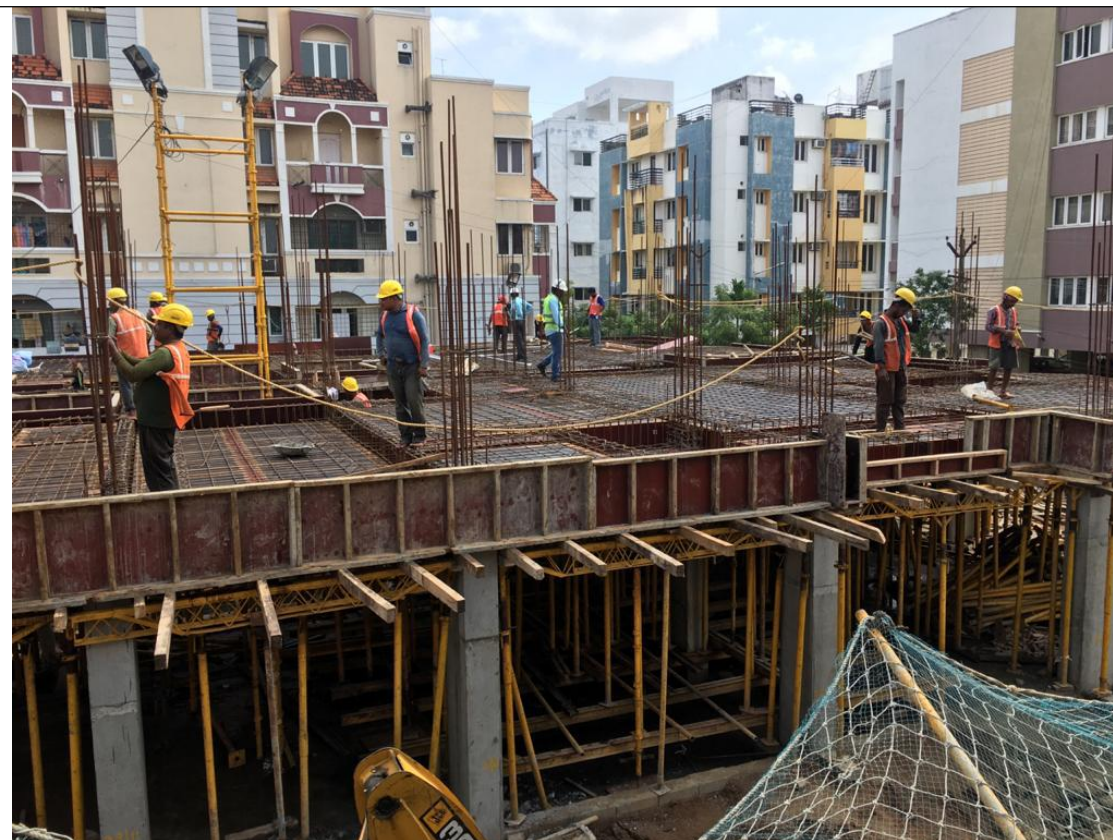
Stilt floor roof slab reinforcement checking(B-2)
