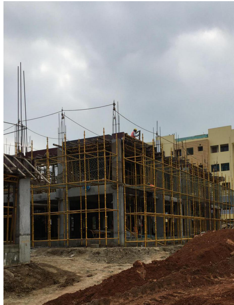
Fig 04 - Safety Net Around Structure
