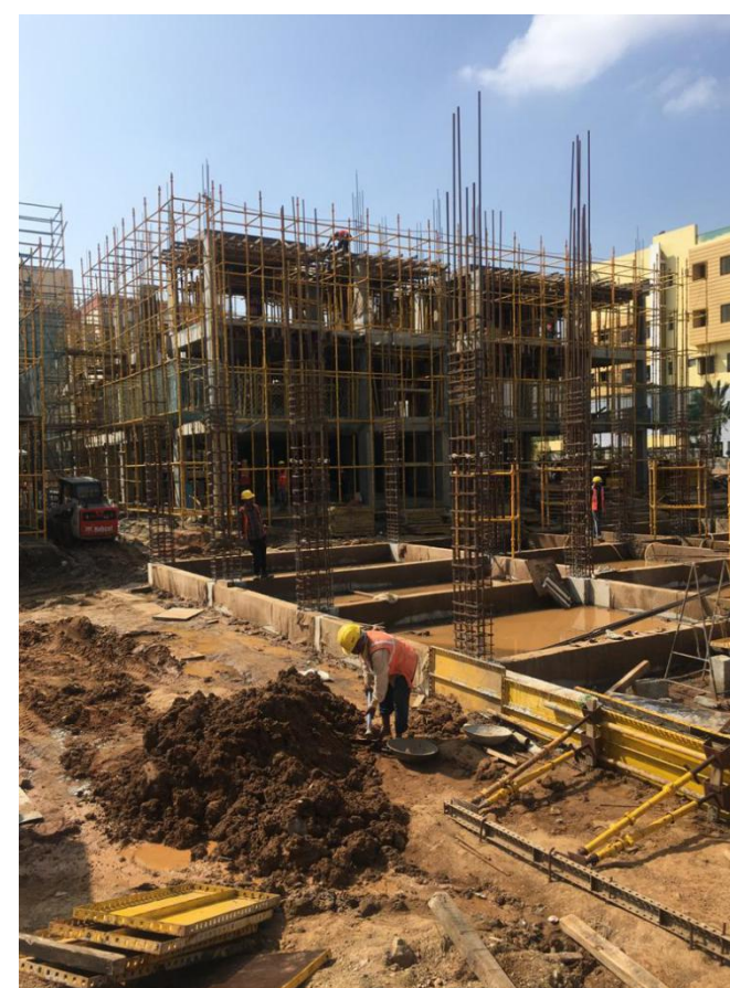
Part plinth beam formwork (B-5)
