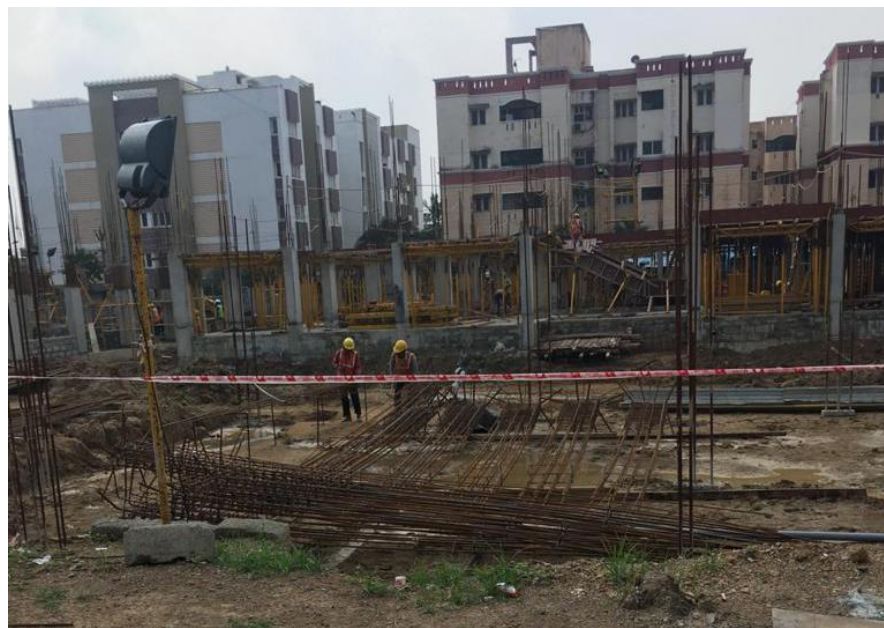
Fig 06 - Tape Barrier around active construction area
