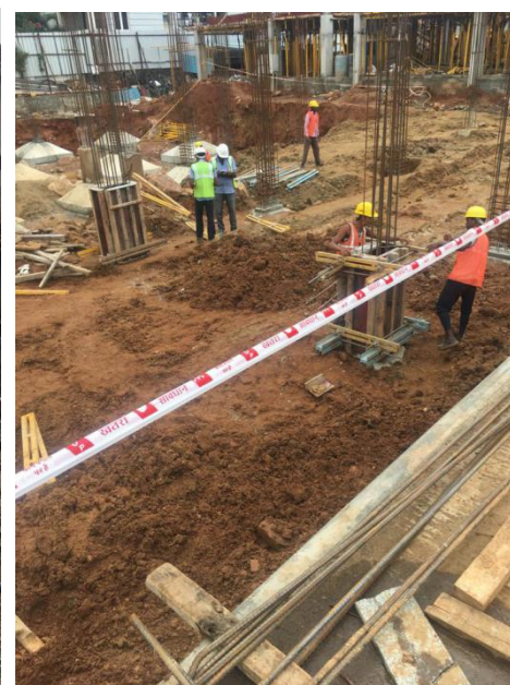
Fig 06 - Tape Barrier around active construction area
