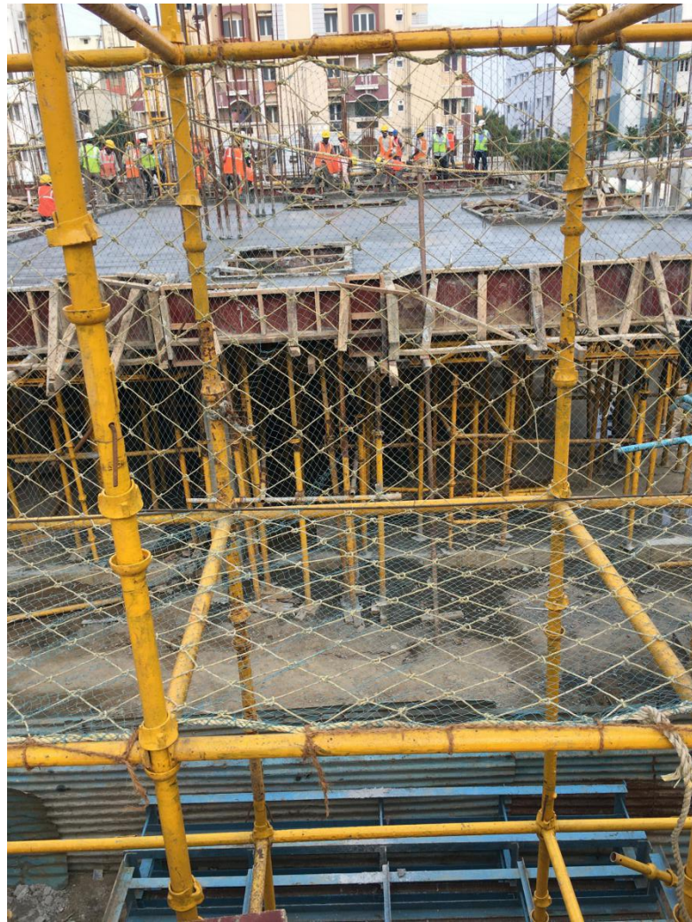
Fig 03 - Safety Net Around Structure
