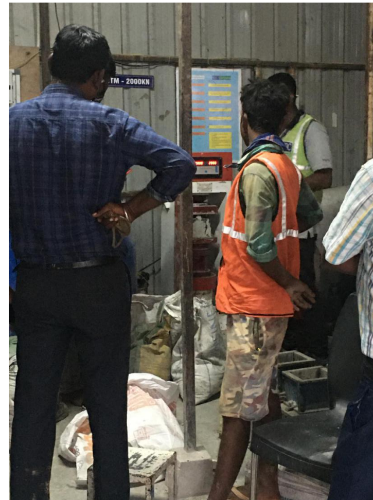
Fig 09 - RMC Mix - Cube Testing at RMC Plant
