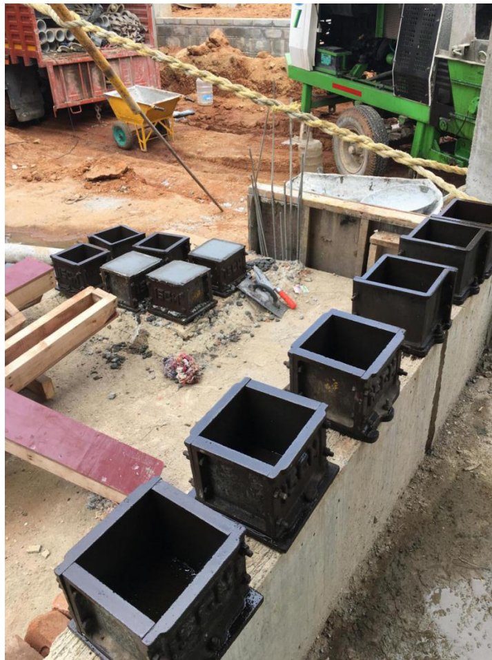
Fig 08 - RMC Mix - Cube Testing Sample making
