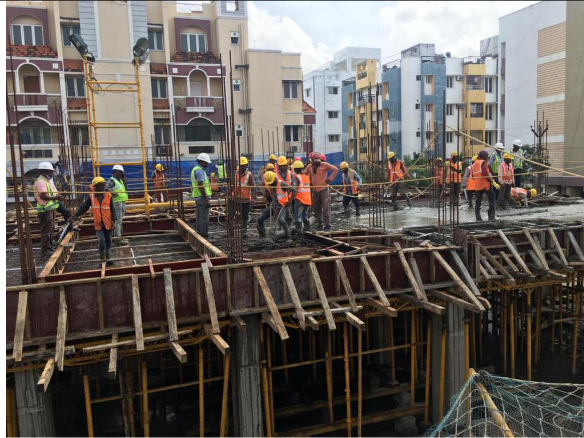
Concreting of Roof slab of stilt floor(B-2)
