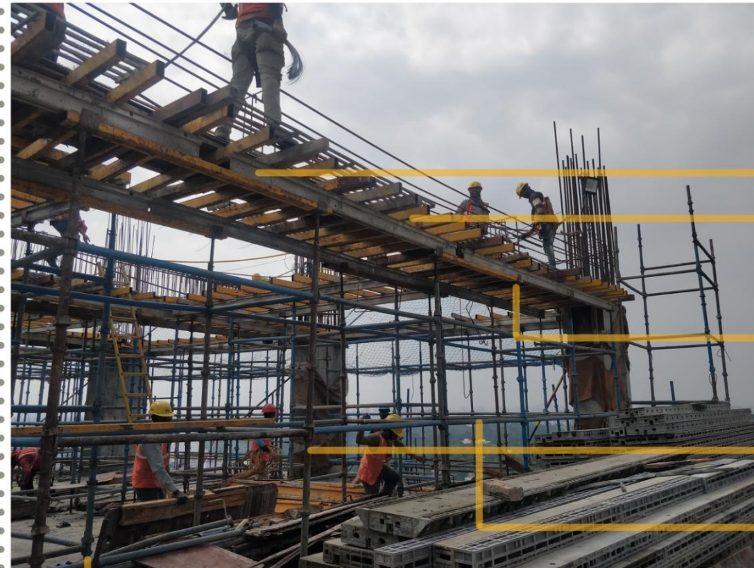
Flat section for scaffolding ledger
