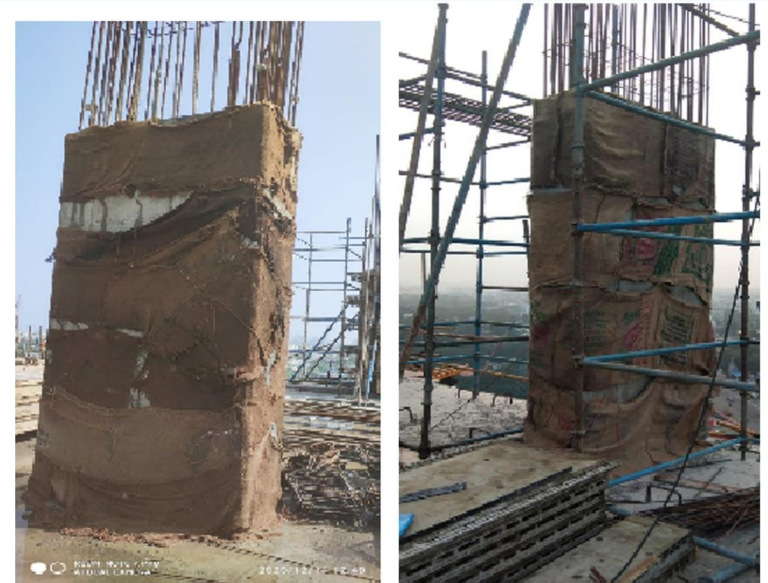
Curing using gunny bags
