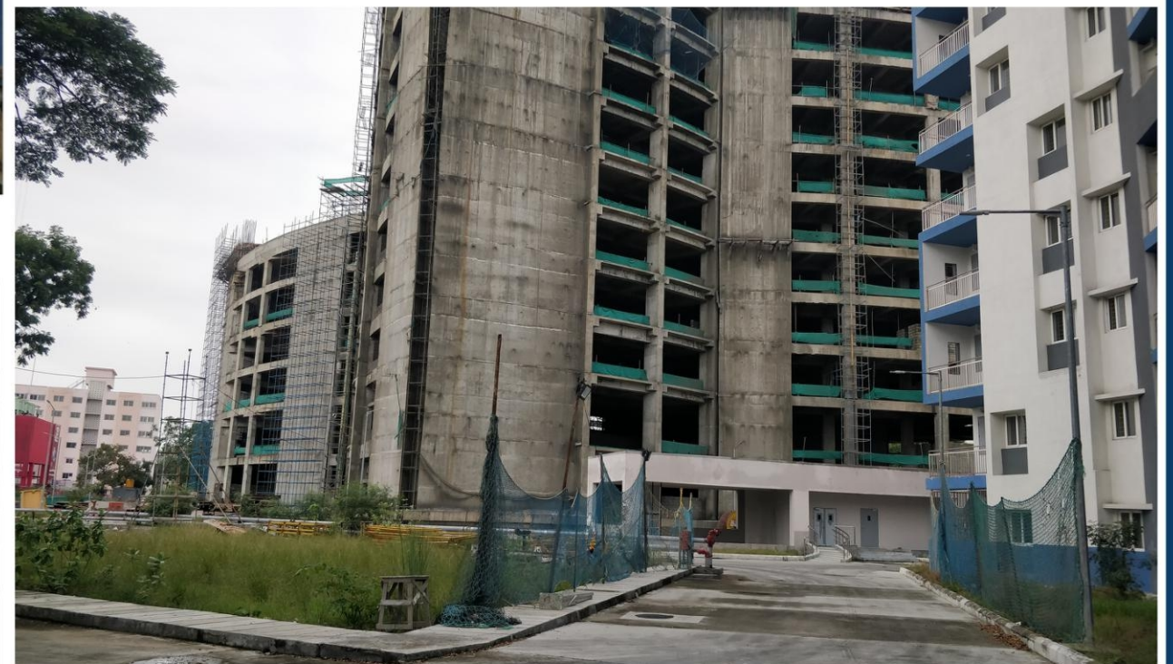
BASEMENT STAIRCASE AND AMENITIY AREA
