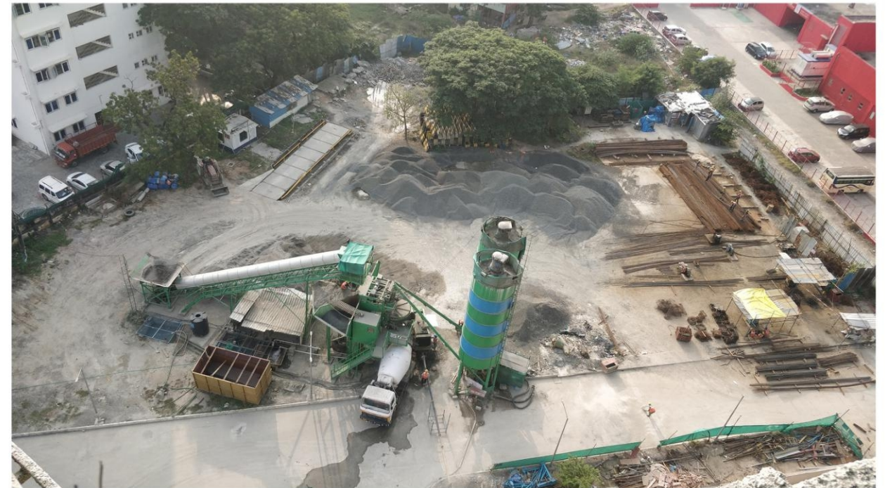
BACTHING PLANT AND STEEL YARD
