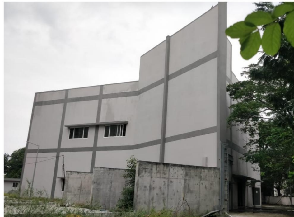
UTILITY BUILDING AND TRANSFORMER
