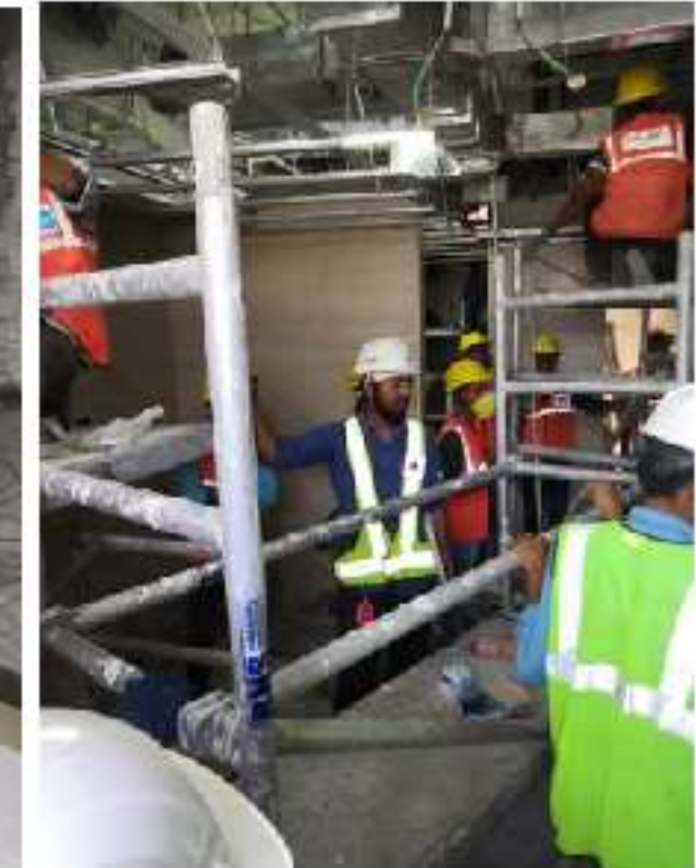
FIXING OF SUPPLY AND EXHAUST AIR DUCT
