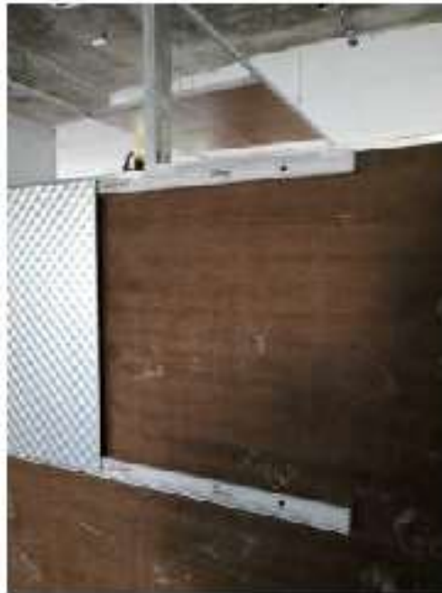
PLY BACKING FOR MIRROR FIXING
