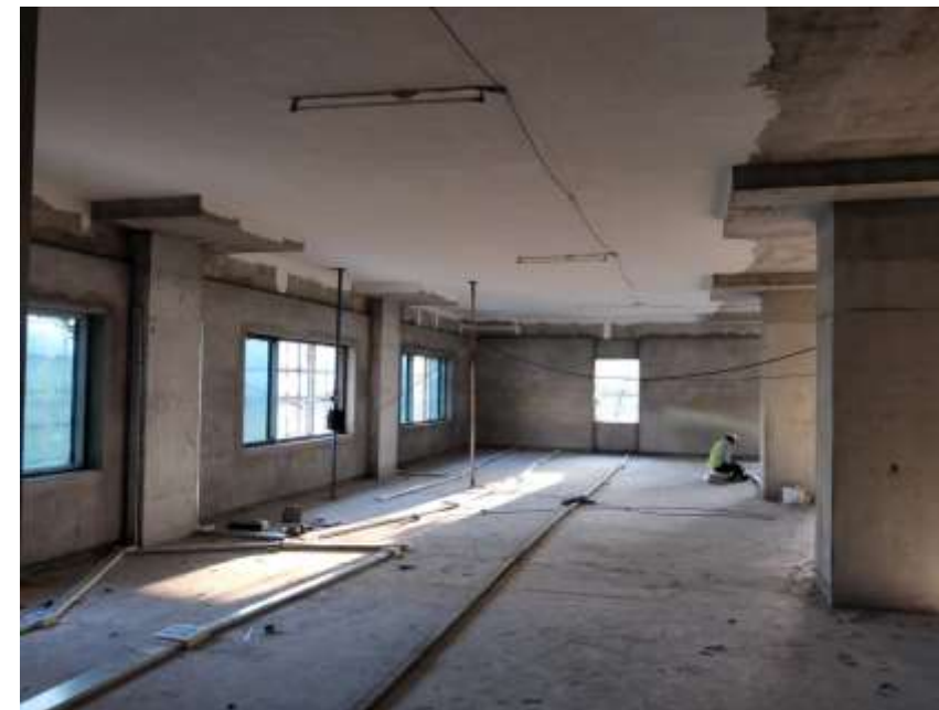
WORK STATION AND COMMON AREAS – OPEN CEILING PUTTY WORK
