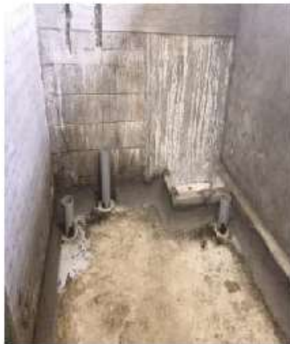
2 ND FLOOR CORE PACKING WORK
