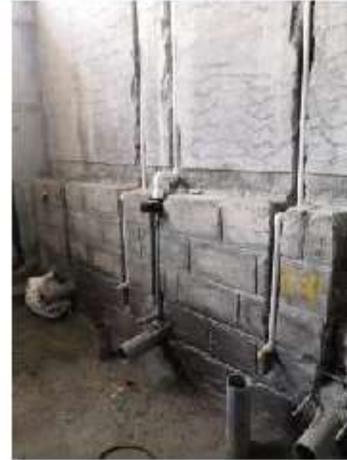
INSERTING SUPPLY AND DRAINAGE LINES
