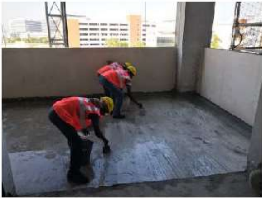
WATERPROOFING PANTRY AREA
