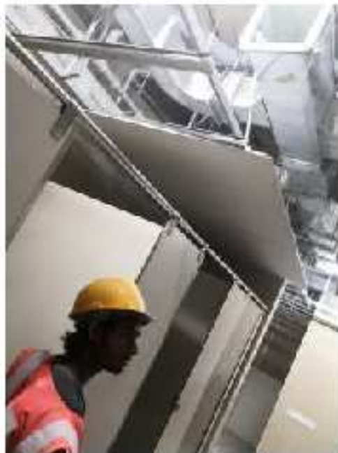
FIXING OF CUBICLE PARTITIONS
