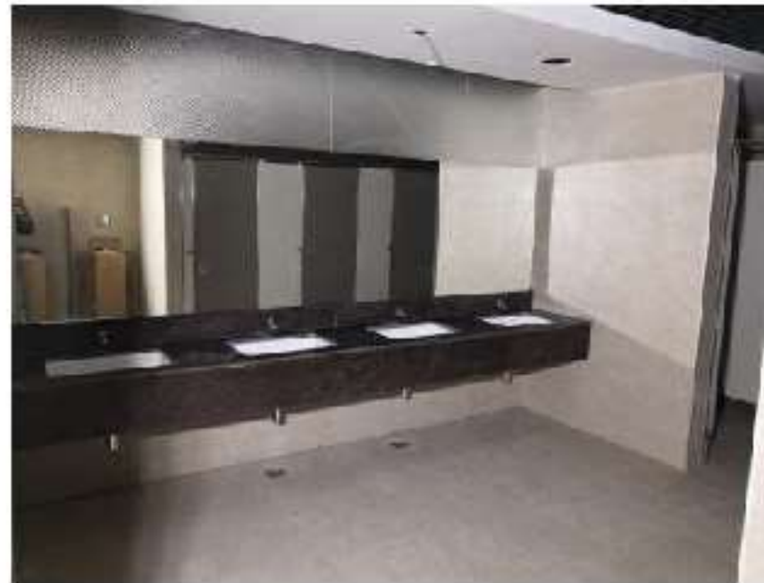
BOXING FOR COUNTER AND GRANITE LAYING
