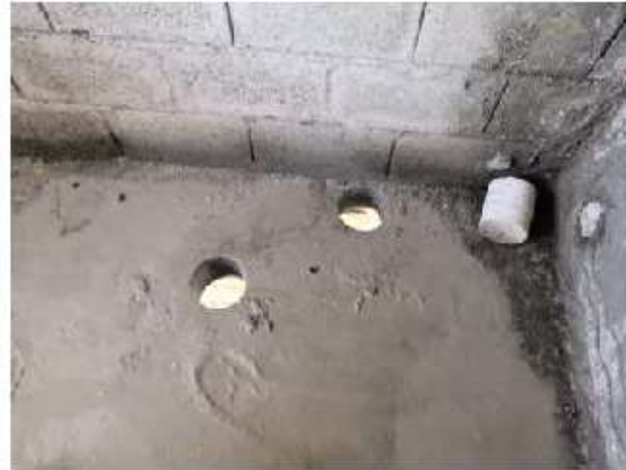
3 RD FLOOR CORE CUTTING WORK
