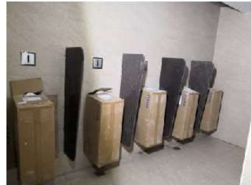
FIXING OF SANITARY FIXTURES
