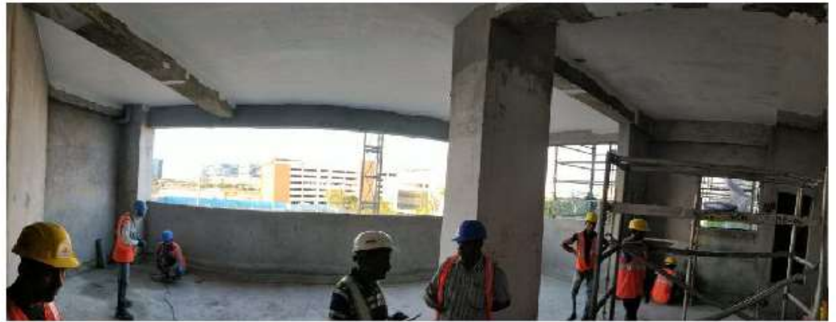
CEILING PUTTY WORK
