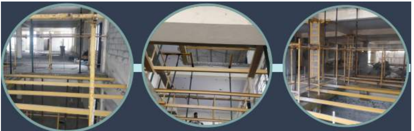
Fig:4.2.5: Current condition of the building
