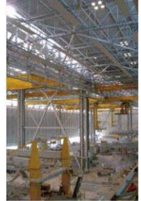
Fig 1 Internal view of the building during construction
