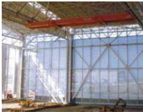
Fig 3 Roof and roof trusses
