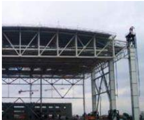
Fig 2 Roof and roof trusses
