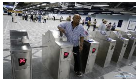
Fig 1.2 AUTOMATIC FARE COLLECTION SYSTEM - AFC
