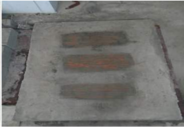
Fig 2.9 - Curing of the Slab
