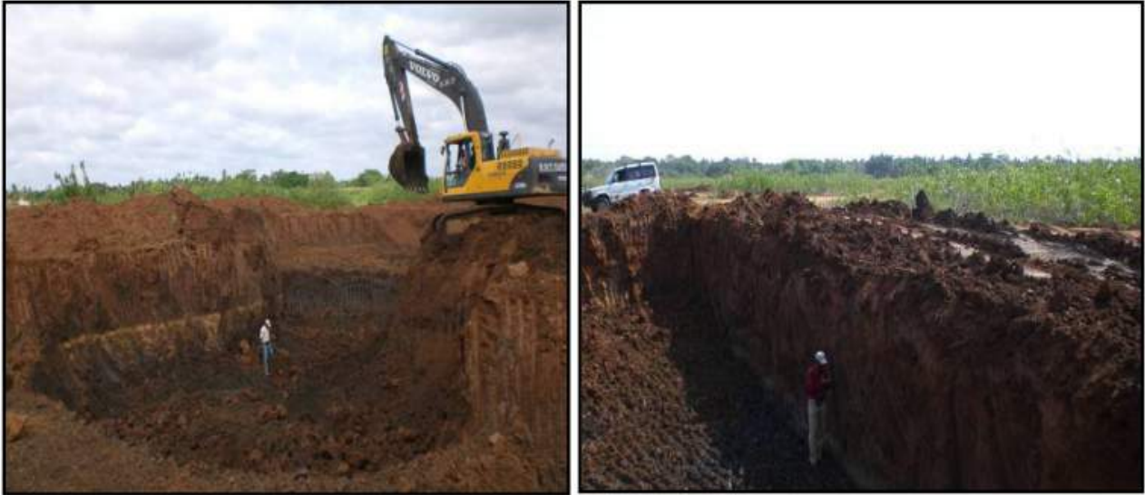
Fig 2.10 - Clay Excavation Process
