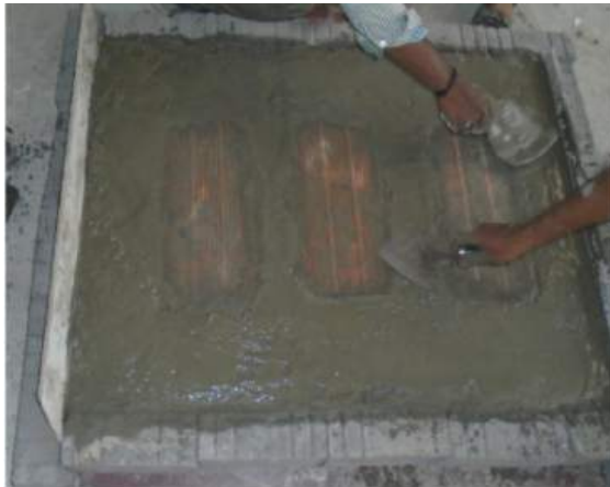
Fig 2.7 - Casting of the Concrete Slab
