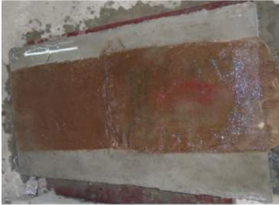
Fig 2.8 - Concrete Slab after 1 Day
