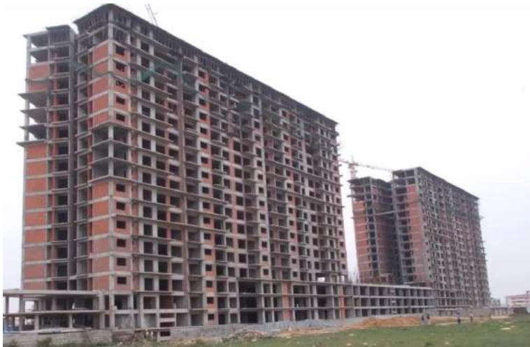
Fig 1.1 - On going High-rised Porotherm Constructed building in Chennai
