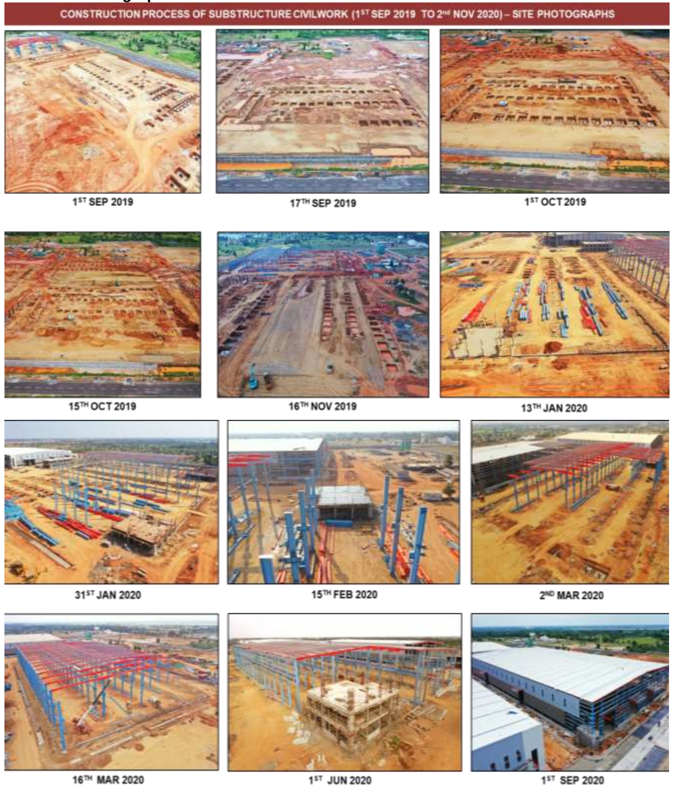
Fig 3.10 Overall Construction Process
