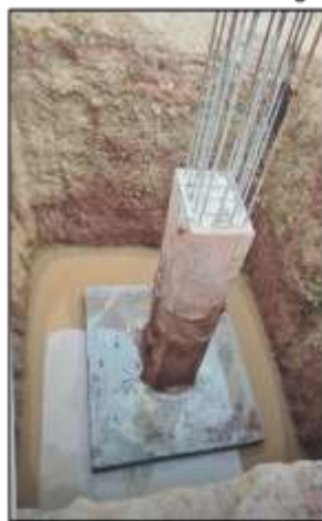
RCC Bldg Pedestal-Concreting
