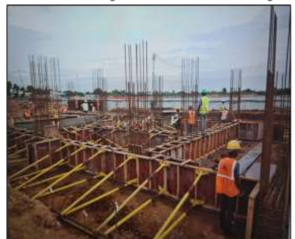
Plinth Beam- Shuttering & Concreting
