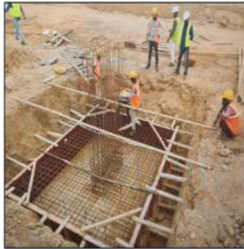
Footing-Rebar work Process
