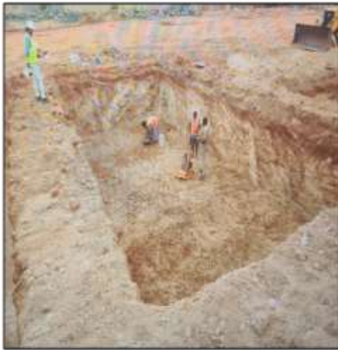
Footing-Excavation Process
