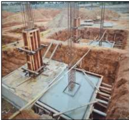
RCC Bldg Pedestal-Shuttering & Concreting
