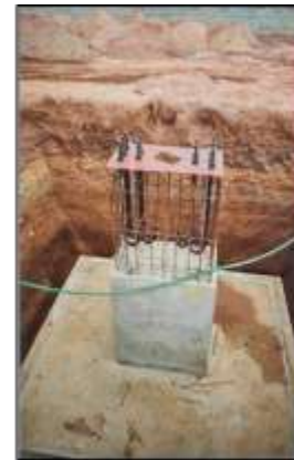
PEB Pedestal 2 nd Lift Bolt Fixing
