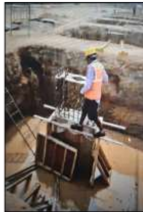
PEB Pedestal 1 st Lift - Concreting
