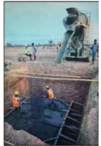
Footing-Concreting Process
