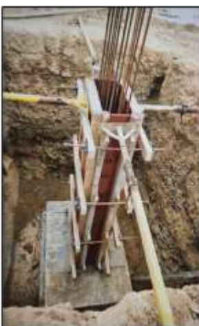
RCC Bldg Pedestal-Shuttering
