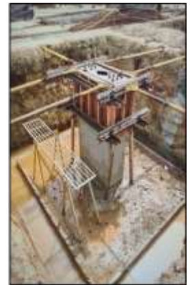
PEB Pedestal 2 nd Lift - Concreting
