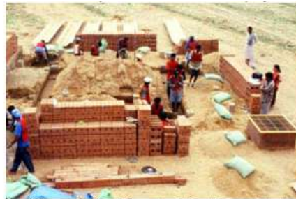
11 hours – Stabilised Rammed earth foundation completed
