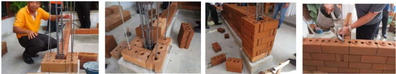
Fig 2.30 Making of Reinforced Column using Interlocking Block (Bredenoord, J., al. Et, 2019)
