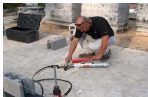
Stage-6: Pre-Stressing the Anchors
