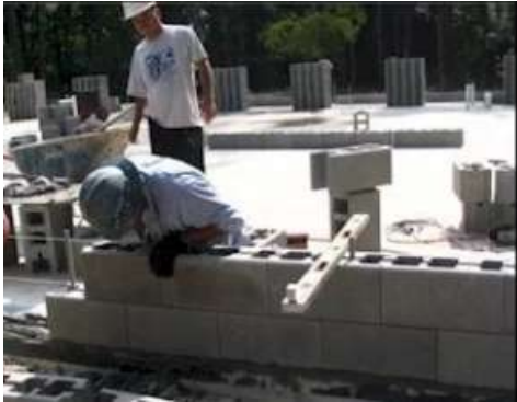
Stage-7: Laying the First Two Courses
