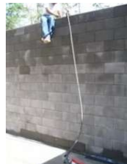
Stage-12: Tensioning the Walls
