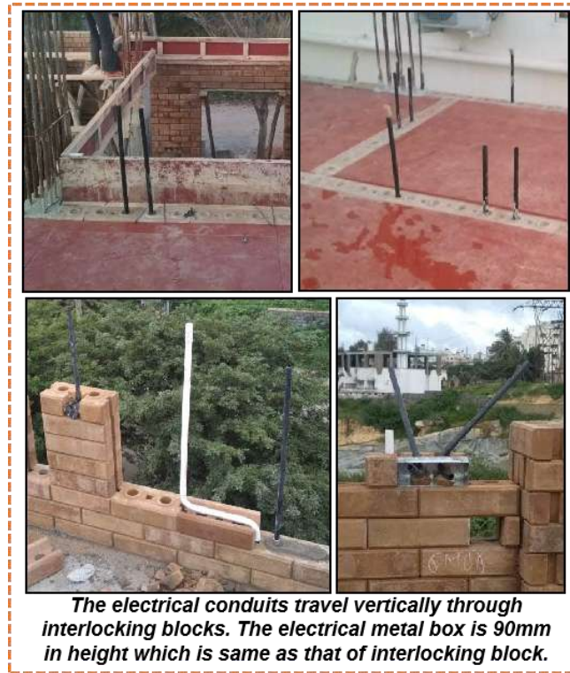
Fig 3.6 Construction Technique of IB MEP Services
