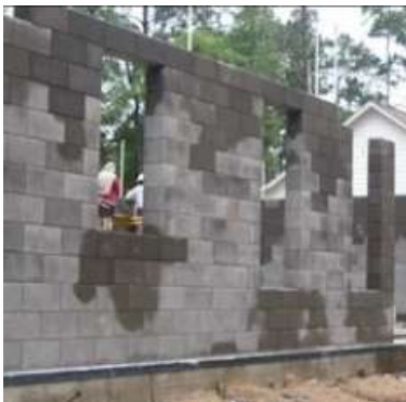
Stage-9: Setting the Lintels
