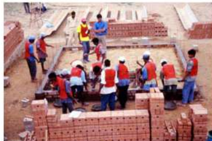
16 hours – Plinth beam completed
