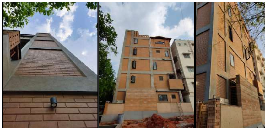
Fig 3.11 Construction Technique - External Plastering
