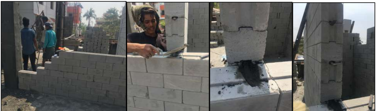
Fig 3.25 Construction Technique - Block Arrangement
