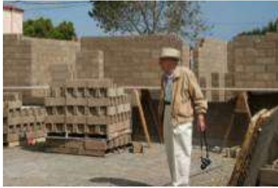
Fig 2.63 Haener House, Napa - Construction
