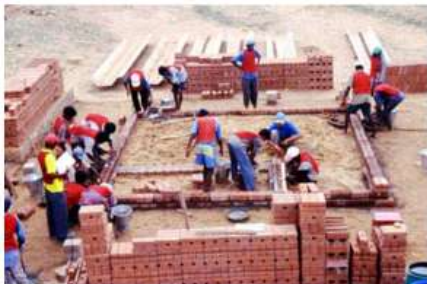
14 hours – Building the second course of the plinth
