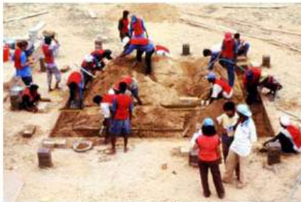
6 hours – Digging the foundations
