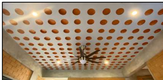
Fig 3.9 Construction Technique - Filler Roof Slab
