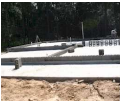
Stage-3: Dry Laying the First Course
