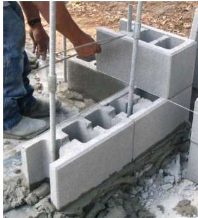
Fig 2.43 First course set in mortar around vertical tendons.
