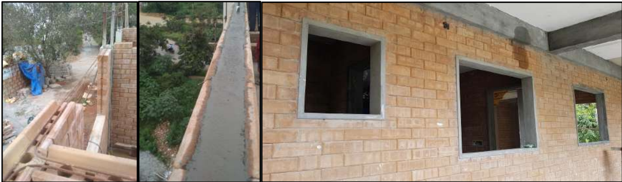
Fig 3.8 Construction Technique of IB - Lintel using U-Block
