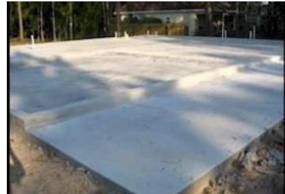
Stage-2: The Finished Slab
