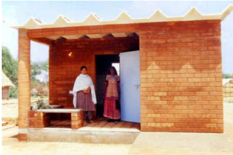
Fig 2.56 AUM House, Gujarat, India - 2001
