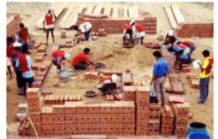
13 hours – Building the first course of the plinth
