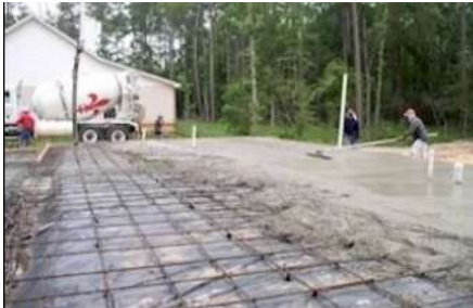
Stage-1: Pouring the base slab
