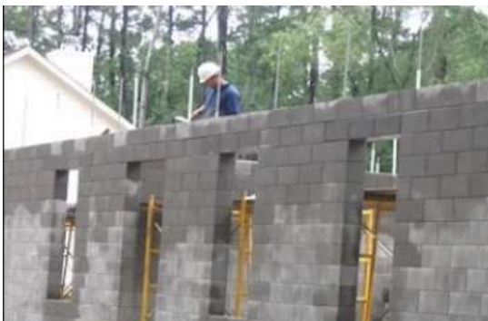
Stage-11: Gouting the Bond Beam
