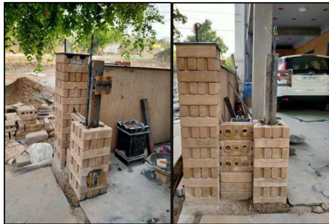
Fig 3.13 Construction Technique - Compound Gate Fixing
