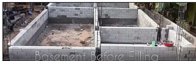
Fig 3.23 Construction Technique - Basement Block Work
