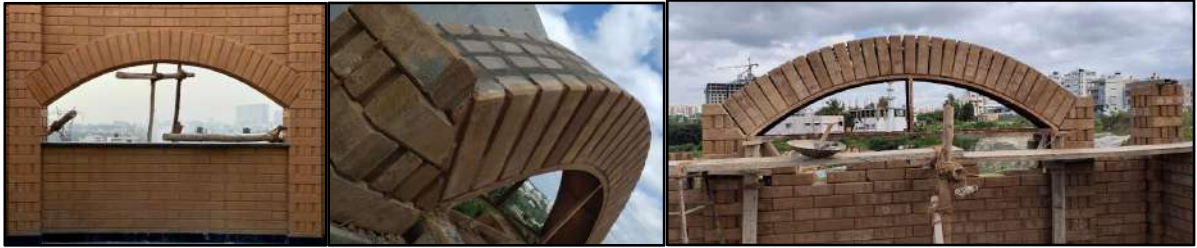
Fig 3.12 Construction Technique - Arch Opening
