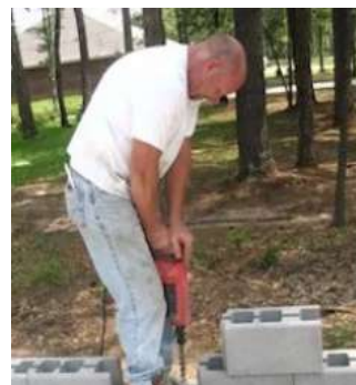
Stage-4: Drilling the Anchor Holes
