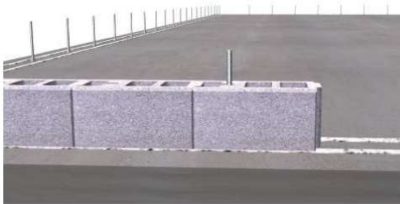
Fig 2.47 Laying of First Course
