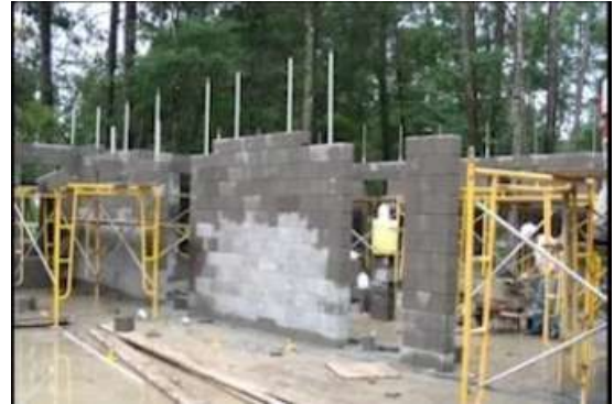
Stage-8: Dry-Stacking the Walls
