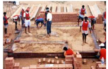
17 hours – Filling the basement and starting the walls
