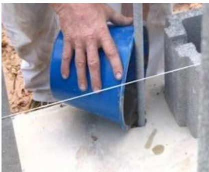
Stage-5: Grouting the Anchors
