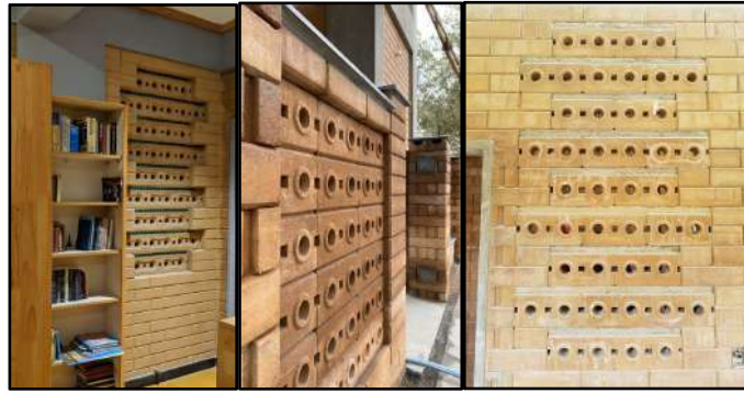
Fig 3.14 Construction Technique - Jalli Wall
