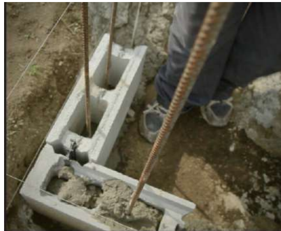
Fig 2.12 The Smart Masonry System - Method (Source- The Smart™ Masonry System)
