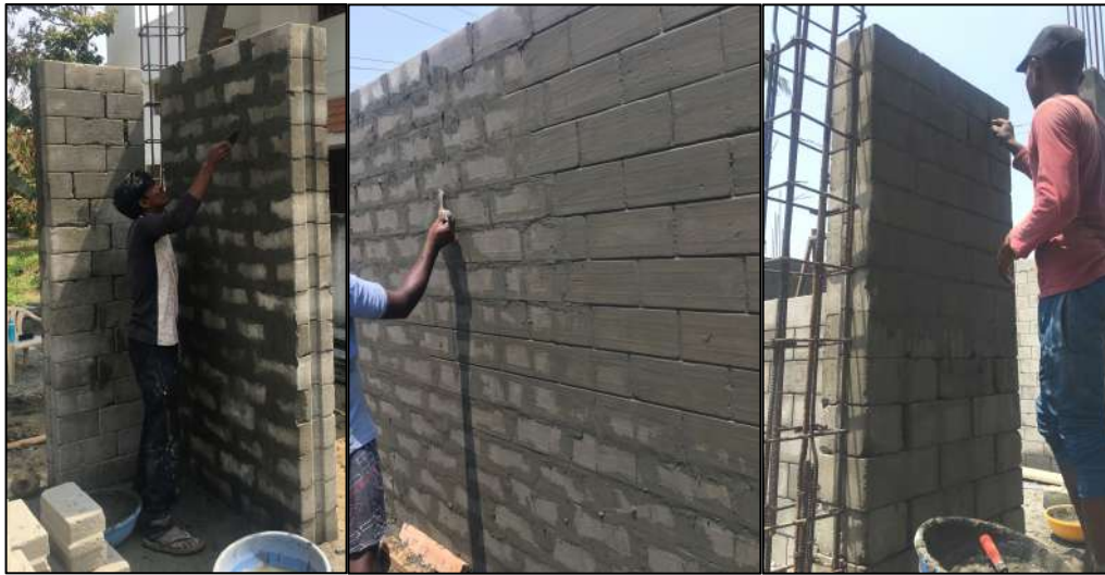
Fig 3.26 Construction Technique - Wall Finishing
