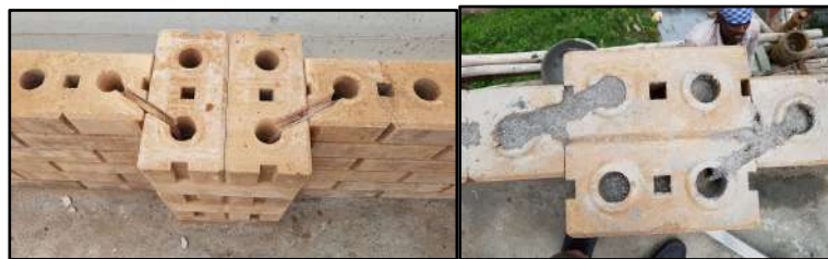
Fig 3.7 Construction Technique of IB Wall Connections
