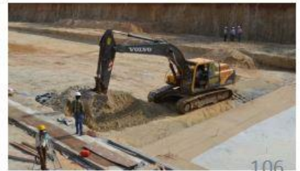
EXCAVATE FOR FOUNDATION
