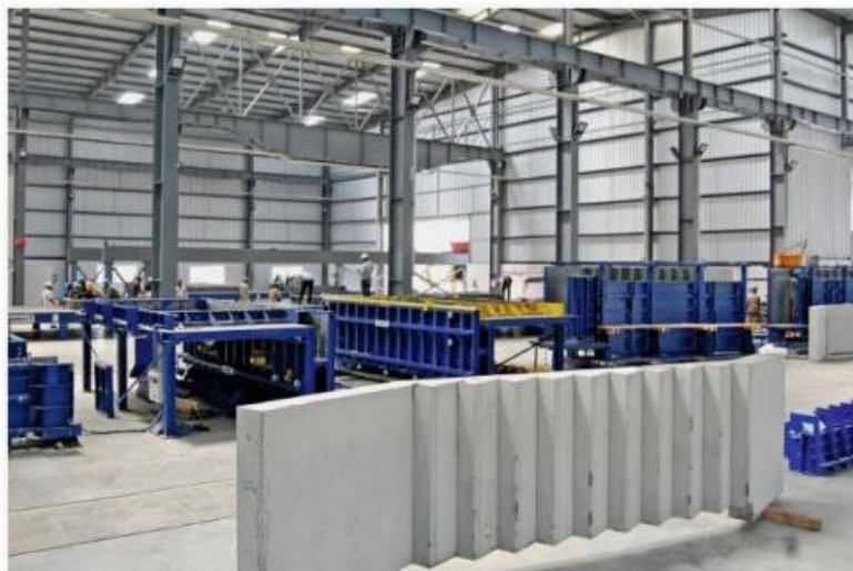
To assure that the entire production process runs at high cycle speed, special components with stationary formwork system are produced by Nuspl, the formwork specialists Figure: Vollert
