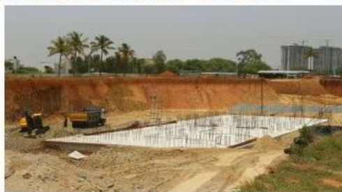
PLINTH BEAM- REINFORCEMENT
