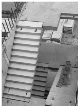
Figure 2.27 – Precast Staircase
