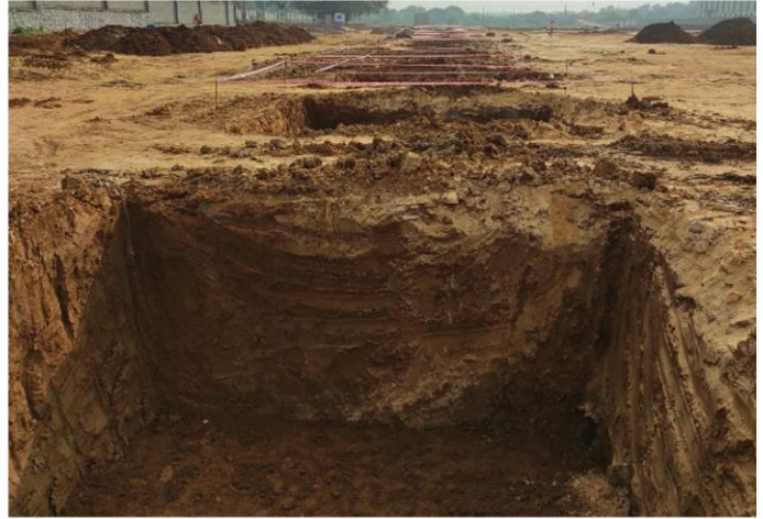
Footing Excavation Work
