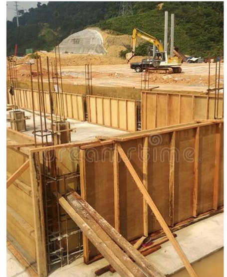
Plywood Formwork
