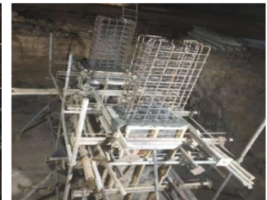
Pedestal 1 st Lift Starter & Concreting Work
