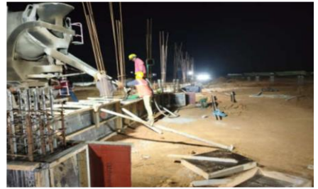
Grade Beam Shuttering & Concreting Work
