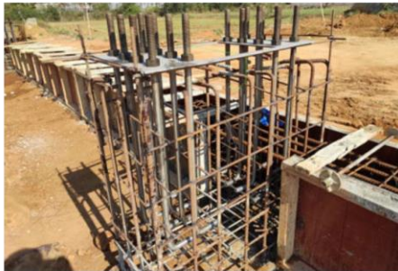
Pedestal Anchor Bolt Fixing
