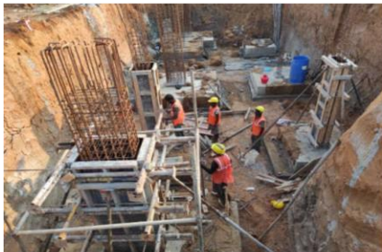
Pedestal Shuttering Work
