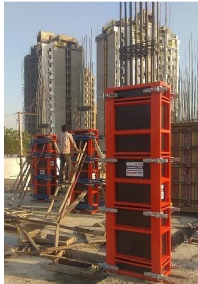
Steel Formwork
