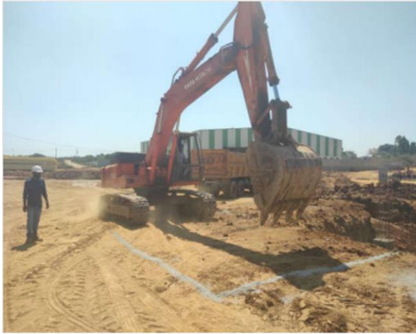
Footing Excavation Work
