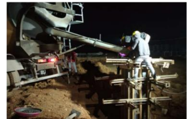
Pedestal 2 nd Lift Concrete Work
