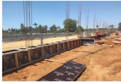
Grade Beam Shuttering & Concreting Work
