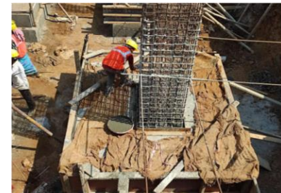
Pedestal 1 st Lift Starter & Concreting Work
