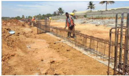
Grade Beam Rebar Work
