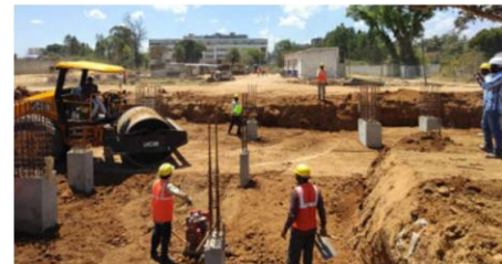
Soil Filling & Compaction Work
