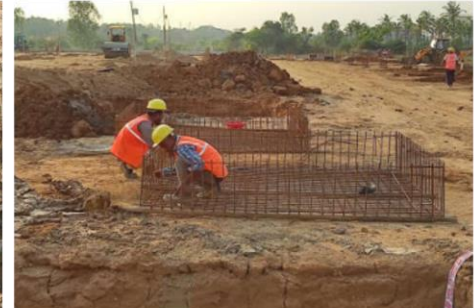
Footing Rebar Work
