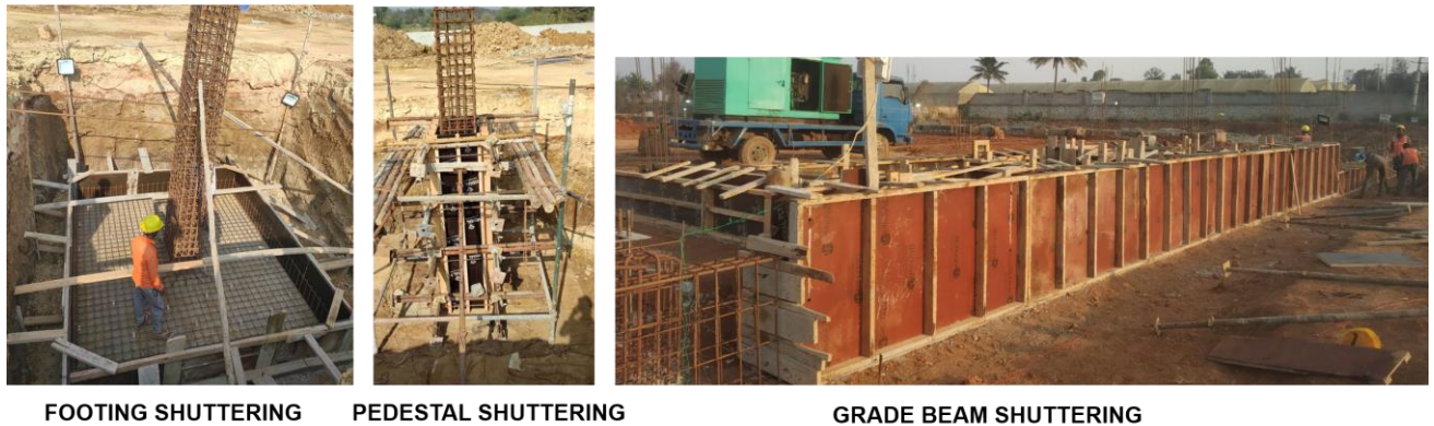
Figure 4.9 Timber Formwork
