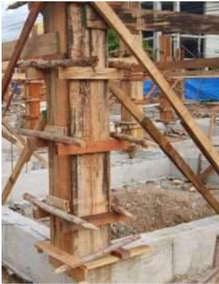
Timber Formwork
