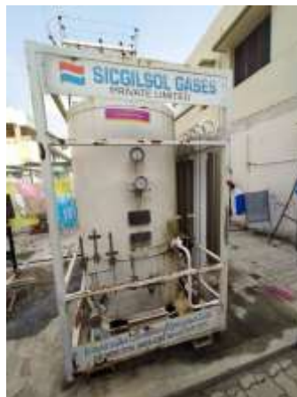
Fig 2.21 Kauvery Hospital Liquid Oxygen Cylinder
