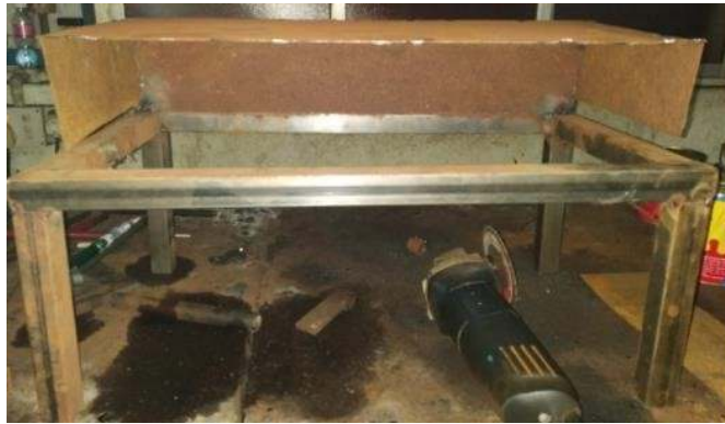
Fig 4.12 Fabrication Attaching the sheet metal to the rectangular frame
