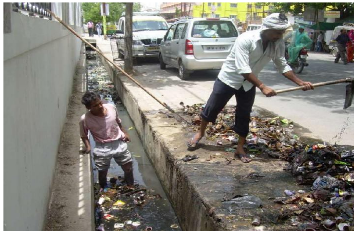
Fig1.1:Manual drainage scrap cleaning
