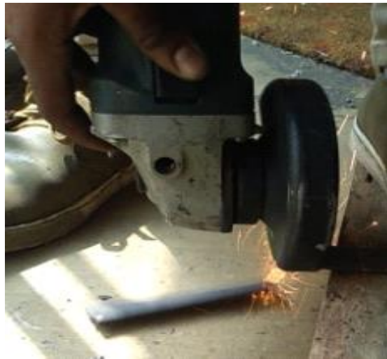
FIG 4.35 CUTTING OF ARM @ 125 MM
