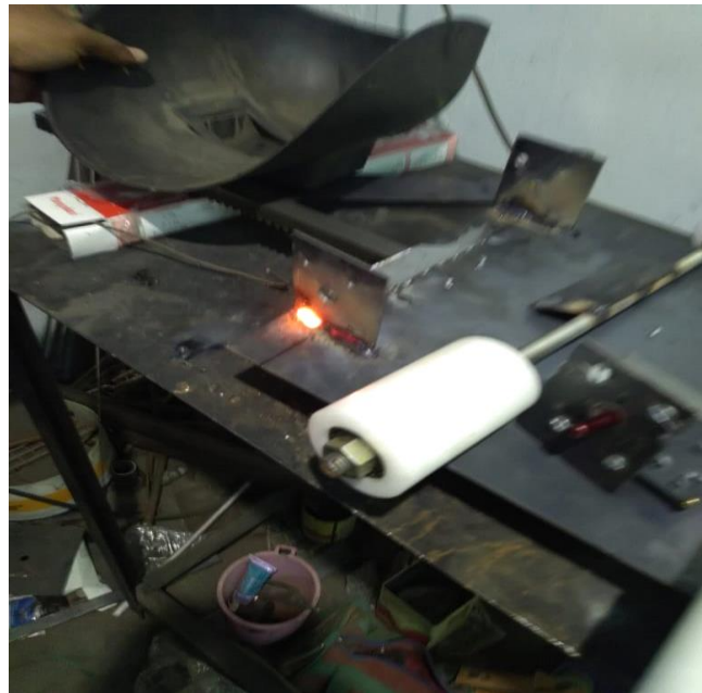
FIG 4.28 VIEW OF WELDING OF MOTOR SUPPORT PLATE TO THE MAIN FRAME
