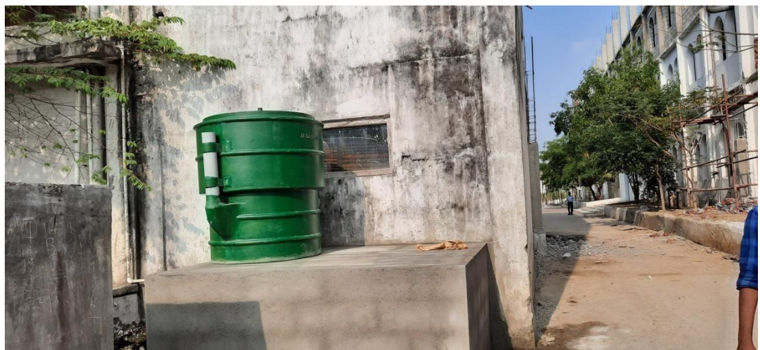
Fig 4.3 installation of plant.
