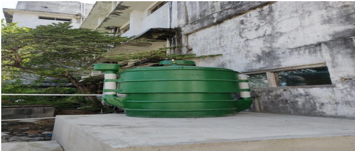
Fig 1.2 Biogas digester tank.
