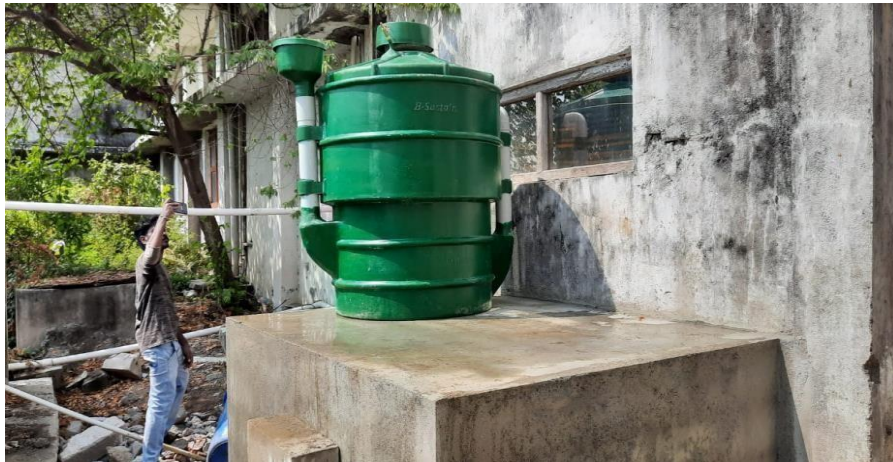
Fig 4.6 Installation of plant is done
