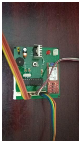
Figure 4.5: voltage regulator was fixed to board
