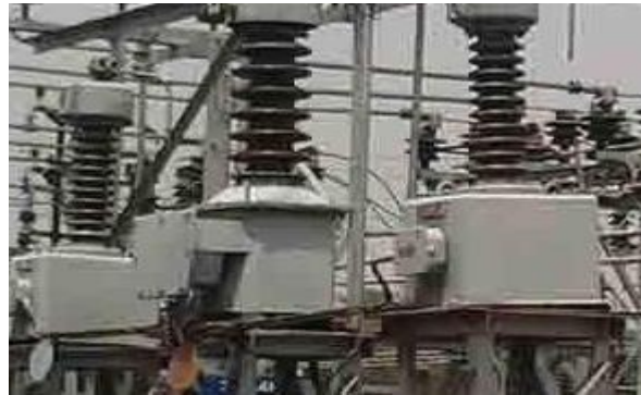
Fig 1.3 : Potential Transformer
