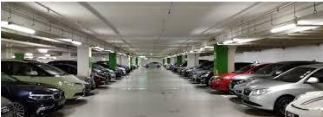
Figure 1.1 Existing Car Parking
