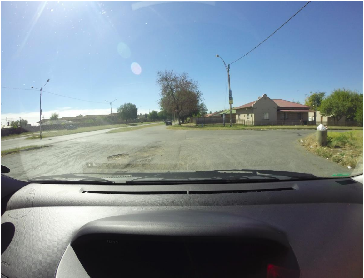
Figure 6.1 Pothole image before predicting
