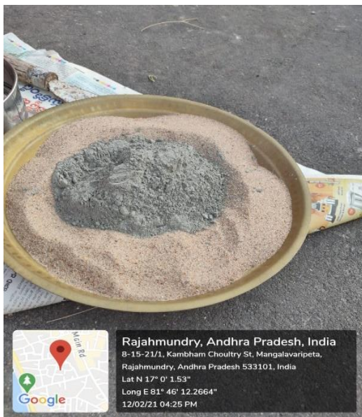
Fig.4.7 Proportioning of cement and sand
