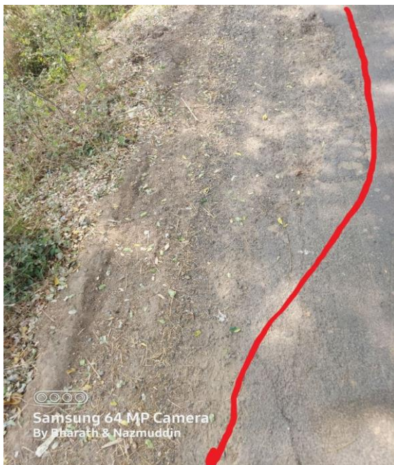
Fig: 4.8: HIGH SEVERITY EDGE CRACKING AT CHAINAGE@1.684KMS
