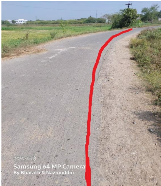
Fig: 4.5: EDGE CRACKING AT CHAINAGE@ 0.105KMS (All dimensions are in meter)
