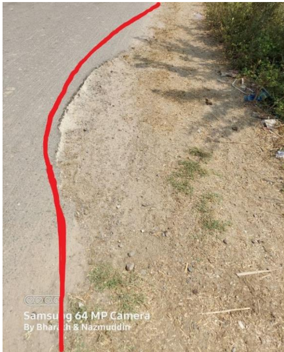
Fig: 4.7: HIGH SEVERITY EDGE CRACKING AT CHAINAGE@0.100KMS
