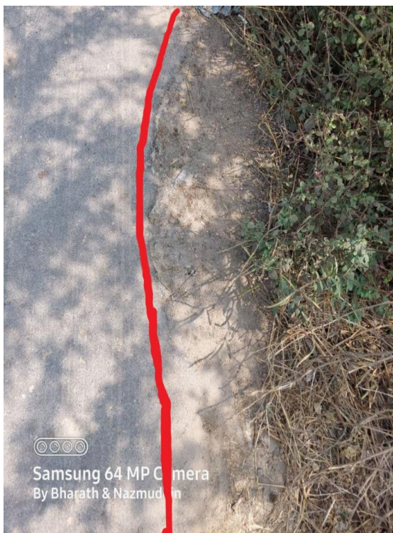
Fig: 4.6: HIGH SEVERITY EDGE CRACKING AT CHAINAGE@0.095KMS
