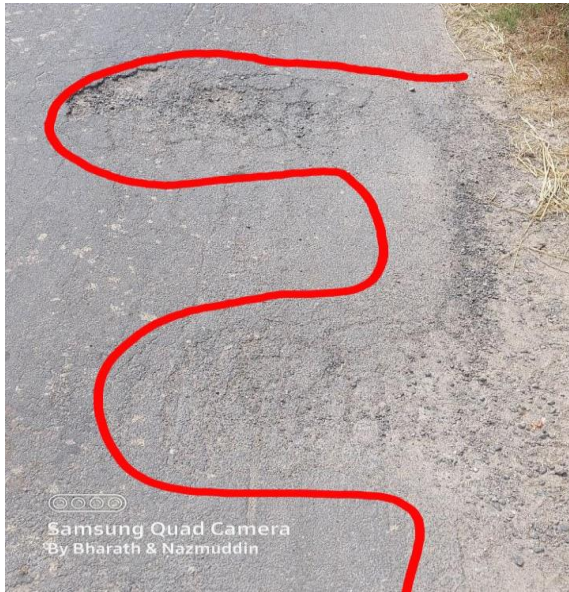
Fig: 4.2: POTHOLE AT CHAINAGE @ 1.721 KMS (all dimensions are in meter)
