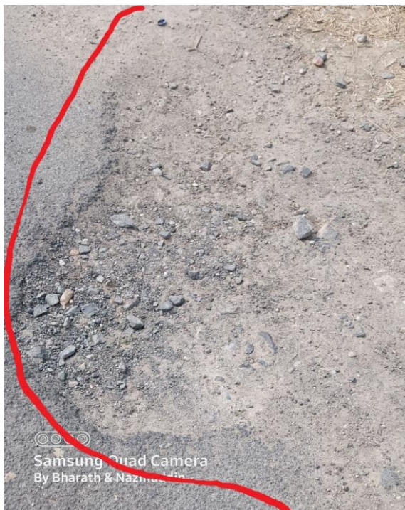
Fig: 4.3: POTHOLE AT CHAINAGE @ 0.973 KMS (All Dimensions Are In Meter)
