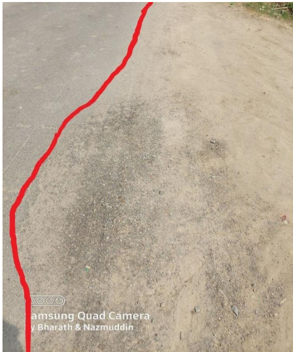
Fig: 4.9: EDGE CRACKING AT CHAINAGE@1.558KMS (All dimensions are in meter)
