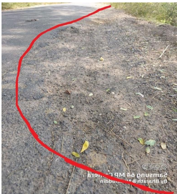
Fig: 4.10: HIGH SEVERITY EDGE CRACKING AT CHAINAGE@0.135KMS (All dimensions are in meter)
