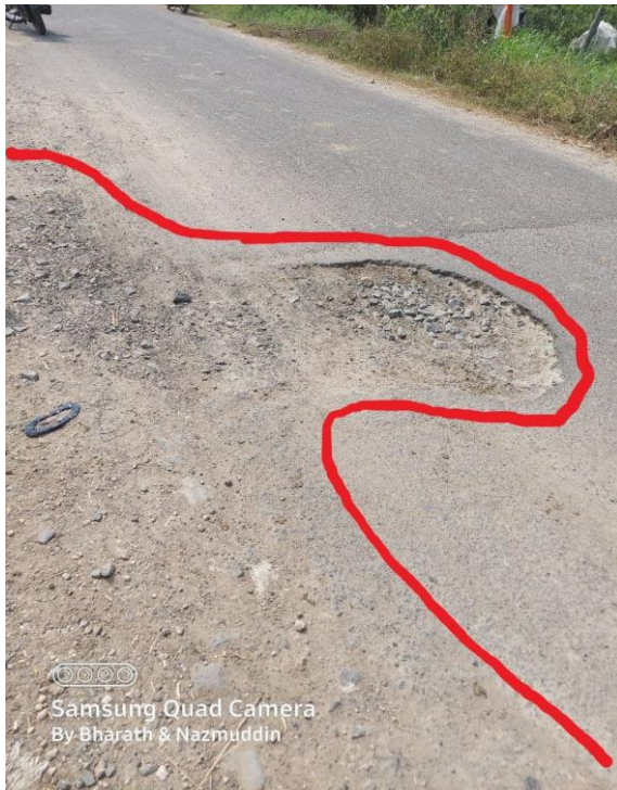
Fig: 4.12: EDGE BREAKING AT CHAINAGE @1.587KMS
