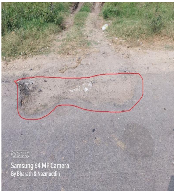
Fig: 4.15: EDGE BREAKING AT CHAINAGE @1.558KMS
