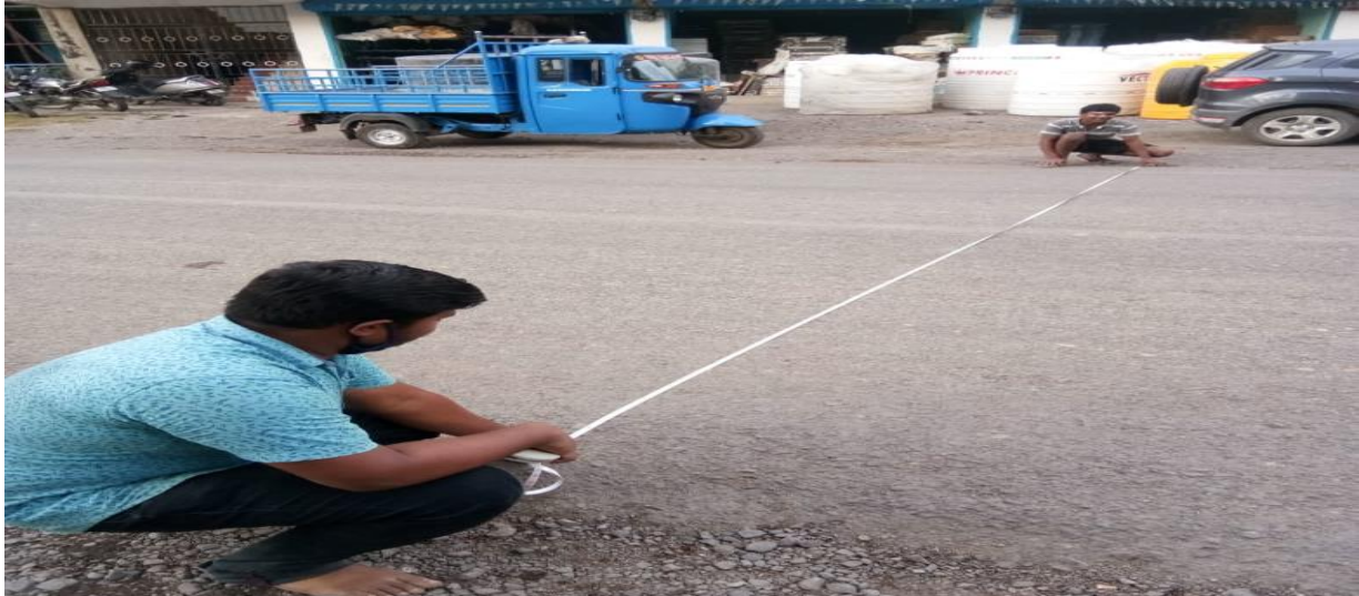
Fig 4.31: Measurement of the width of the Pavement
