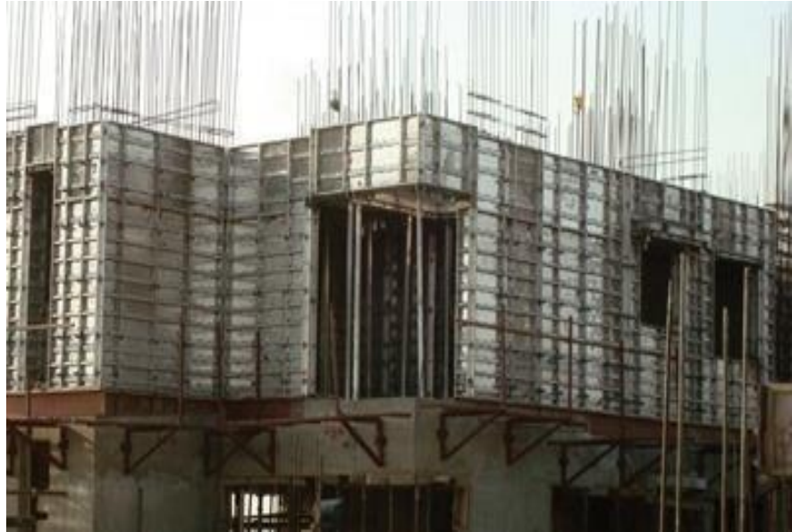
Fig.1.2 Aluminum formwork wall structure
