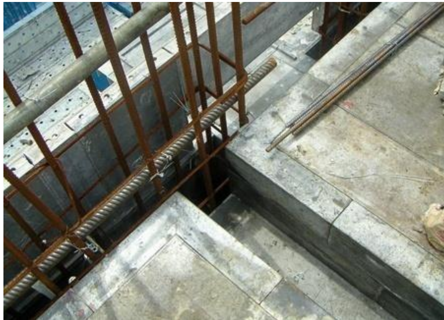
Fig.1.1 Aluminum formwork slab structure
