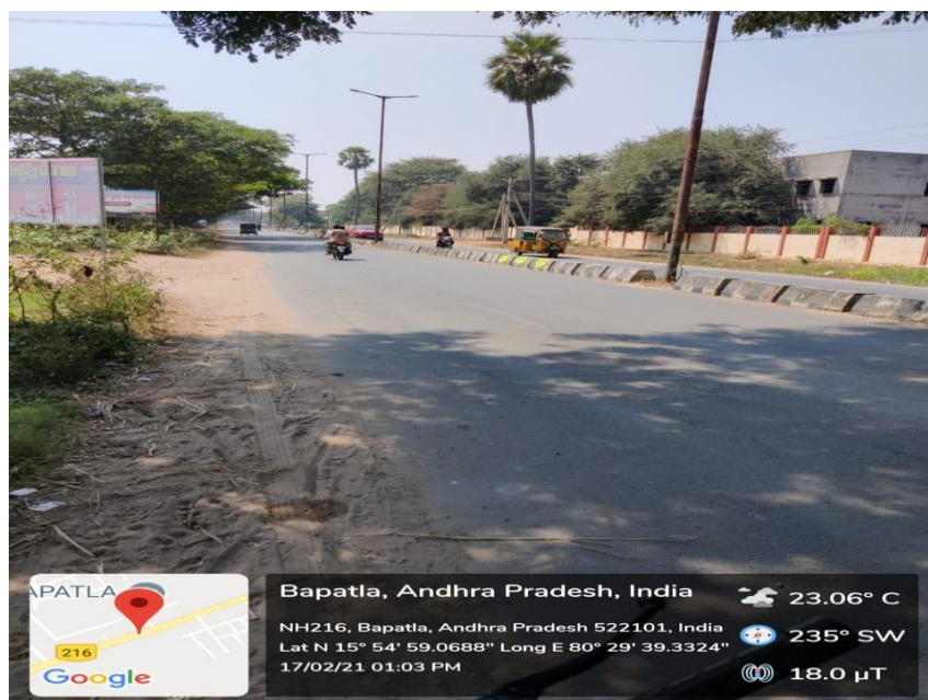
Fig : 3.4 : View of Road Geometry of Arm – A (from market yard) at Bapatla
