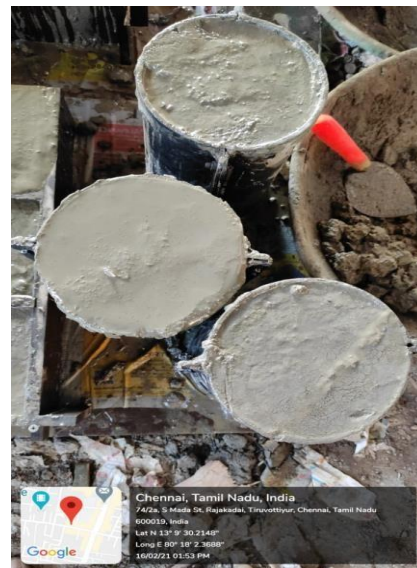
Fig: 4.11 casting of cubes and cylinders
