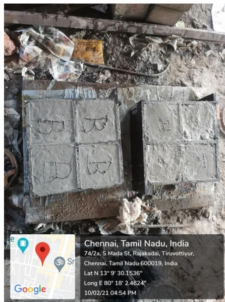
Fig 4.6.2 casting of cubes
