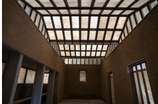
Semi transparent roof, bamboo framework and polycarbonate sheet laid on top.
